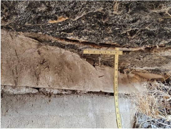
Exposed cross bracing at southeast corner, general
