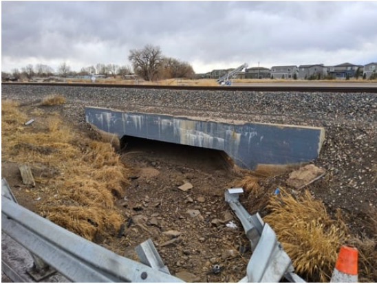
Channel looking south downstream
