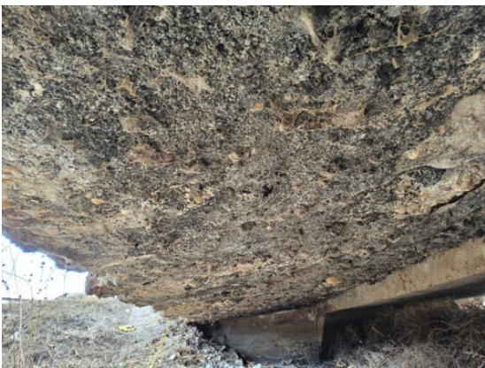
Superstructure looking west
