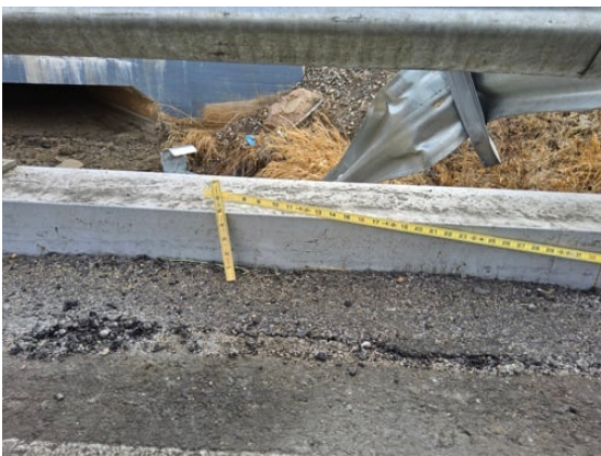
South curb and asphalt wedge at midspan general
