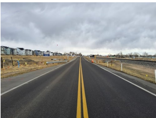
Roadway looking East
