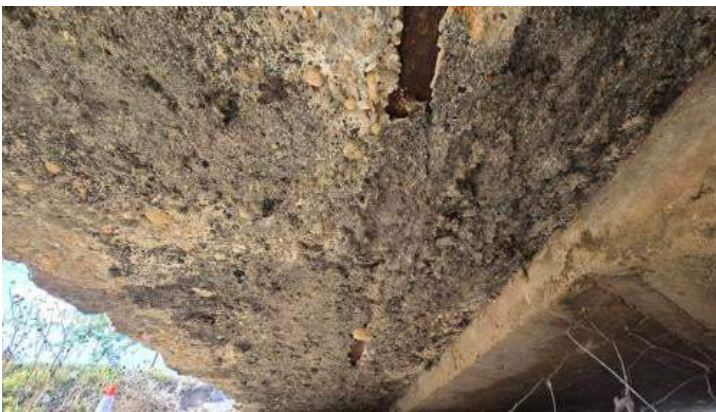
North member bottom flange exposed, general
