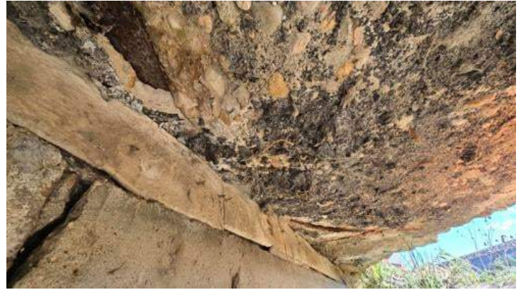
Exposed north member and cross bracing, general
