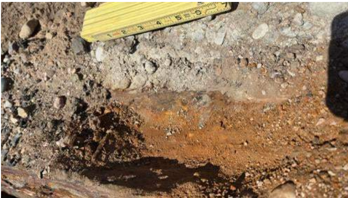
South member upper channel, close-up
