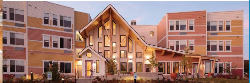
Top left: Second Chance Center's Providence at the Heights (Aurora, CO) | Top right: Brothers Redevelopment Valor on the Fox (Denver, CO) | Bottom: Karis' Laurel House (Grand Junction, CO). All designed by Shopworks Architecture.
