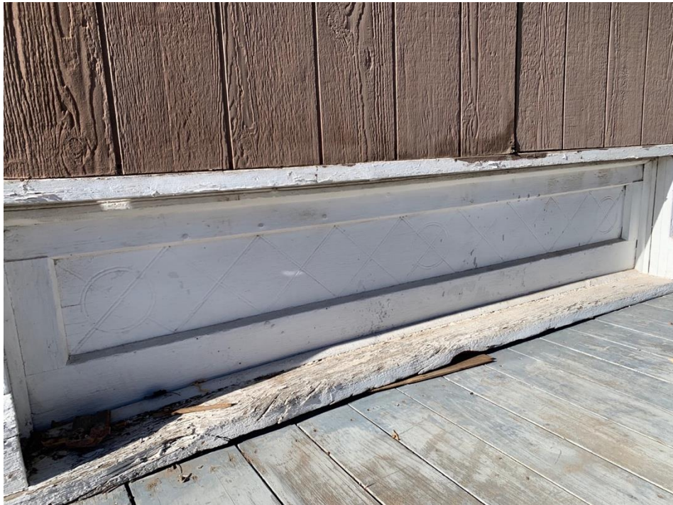
Close-up of the detailed kick-plate on the east elevation of the Emma Malaby Grocery. Photo by Meg Dunn.
