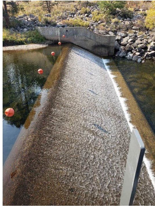
Figure 4-9. Fort Collins Intake at Gateway Park
