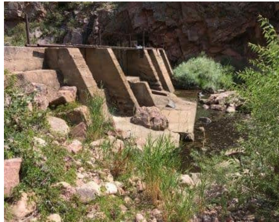
Figure 5-1. North Poudre Canal Diversion Structure
