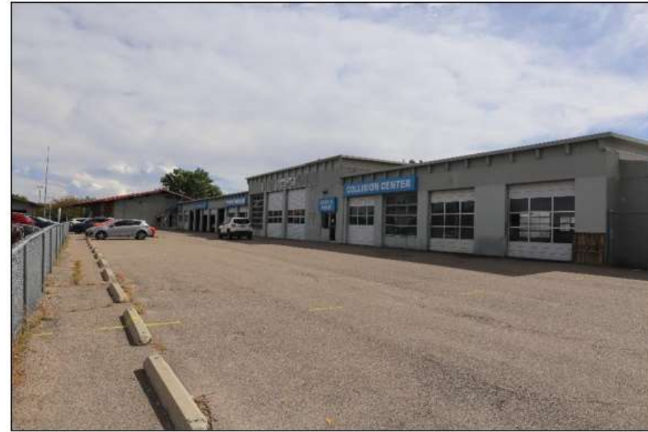
Figure 9: Feature 1, north elevation, view southeast (Image #7229, R. Schields, 10/3/2023)
