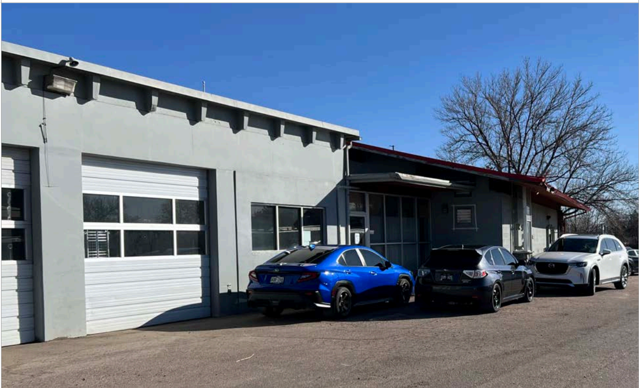
26. West Elevation - Back wall of the Showroom, south portion of elevation. Image courtesy of BEE. 2024.
