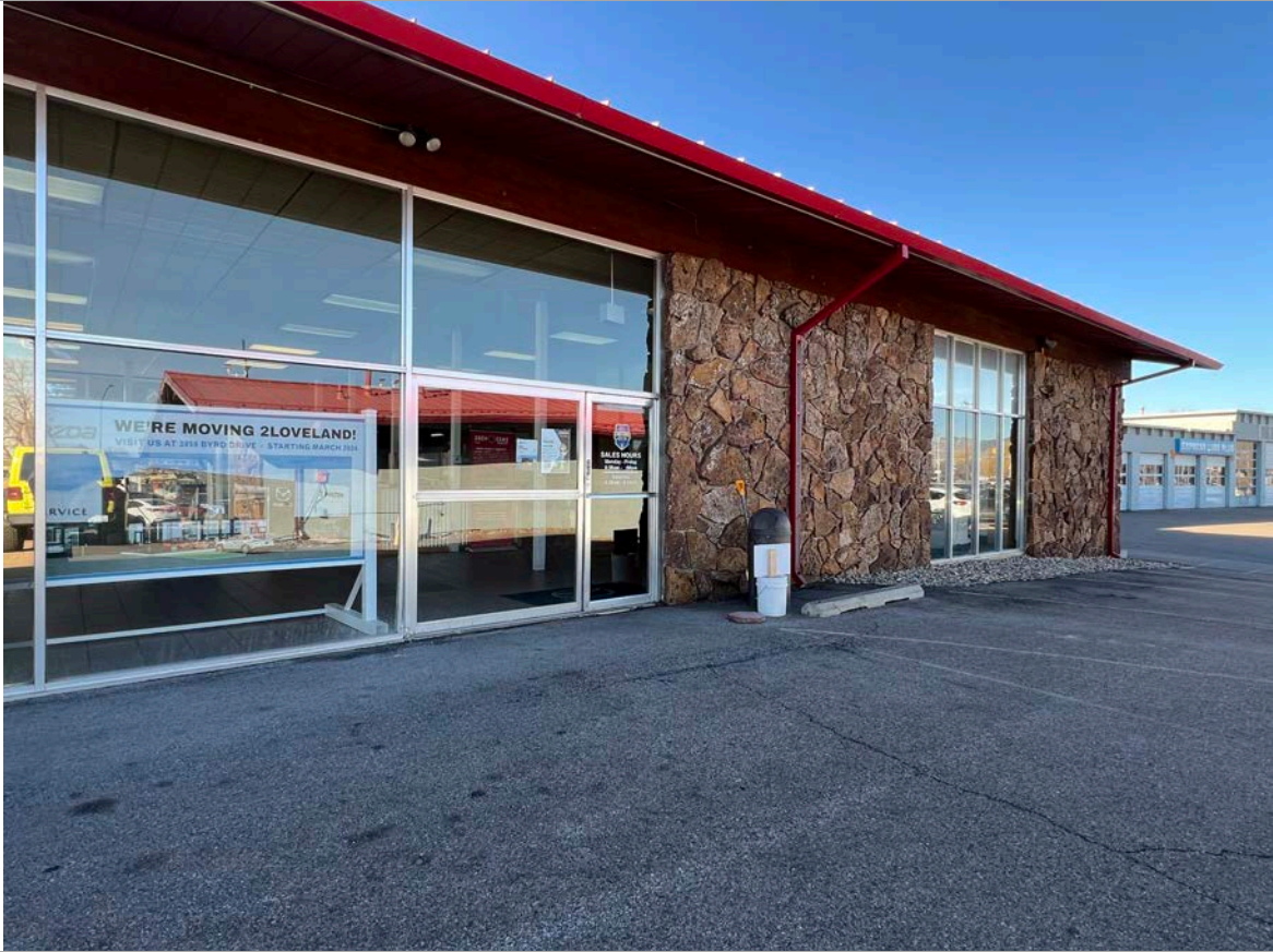
12. North Elevation - of showroom. Note door with hinged window to allow cars into the showroom, located in the middle of the photo frame. Image courtesy of BEE. 2024.
