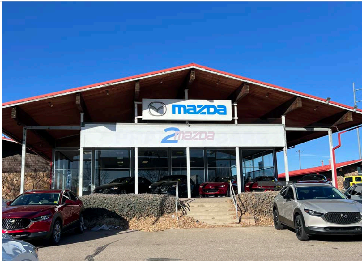
4. East Elevation - North end. Image courtesy of BEE. 2024
