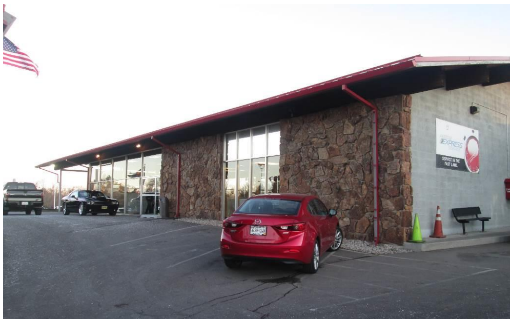
5LR.14283 – Spradley-Barr Showroom (Bldg. A) Northern and western elevations. Looking southwest. December 2017. Image 5LR.14283e.
