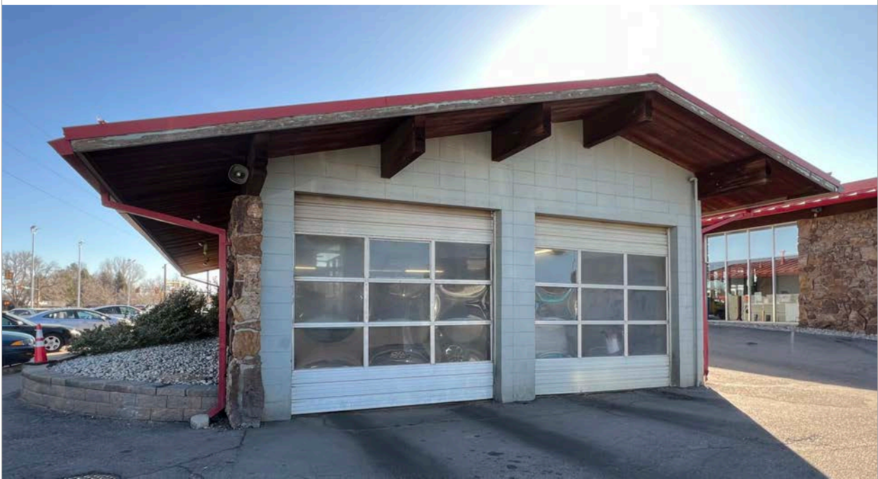
46. West Elevation - Service area with two bays. Image courtesy of BEE. 2024.
