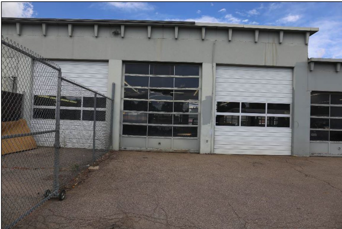
Figure 15: Feature 1, center portion of south elevation, view north (Image #7247, R. Schields, 10/3/2023).
