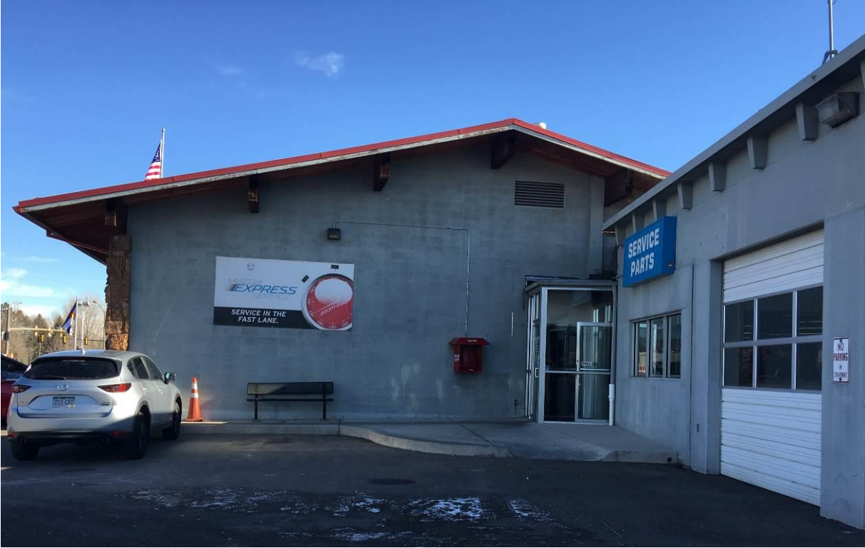
5LR.14283 – Spradley-Barr Parts and Service Entry (Foyer) (Bldg. A) Western elevation. Northern elevation of the Service Bay Section. Looking east. December 2017. Image 5LR.14283g.
