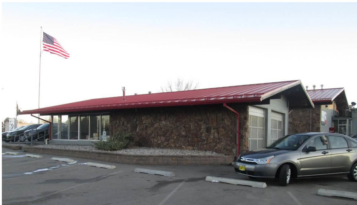
5LR.14283 – Spradley-Barr – Used Car Sales (Bldg. B) Northern elevation. Looking southeast. December 2017. Image 5LR.14283k.
