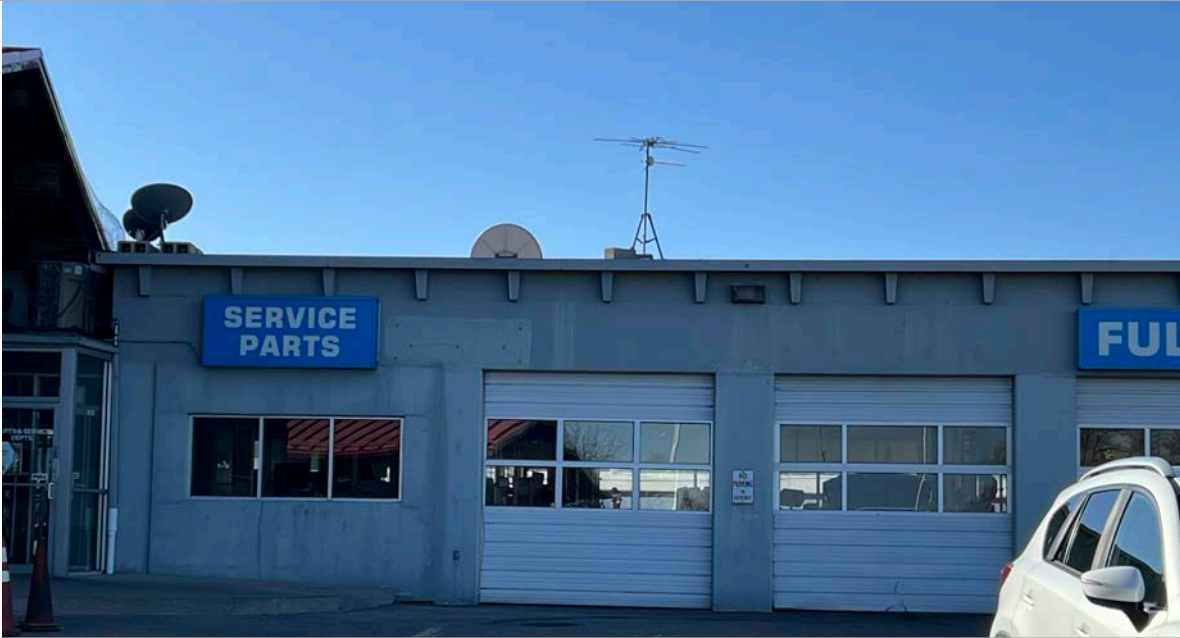
15. North Elevation - Service center, bays 1-2. Image courtesy of BEE. 2024.
