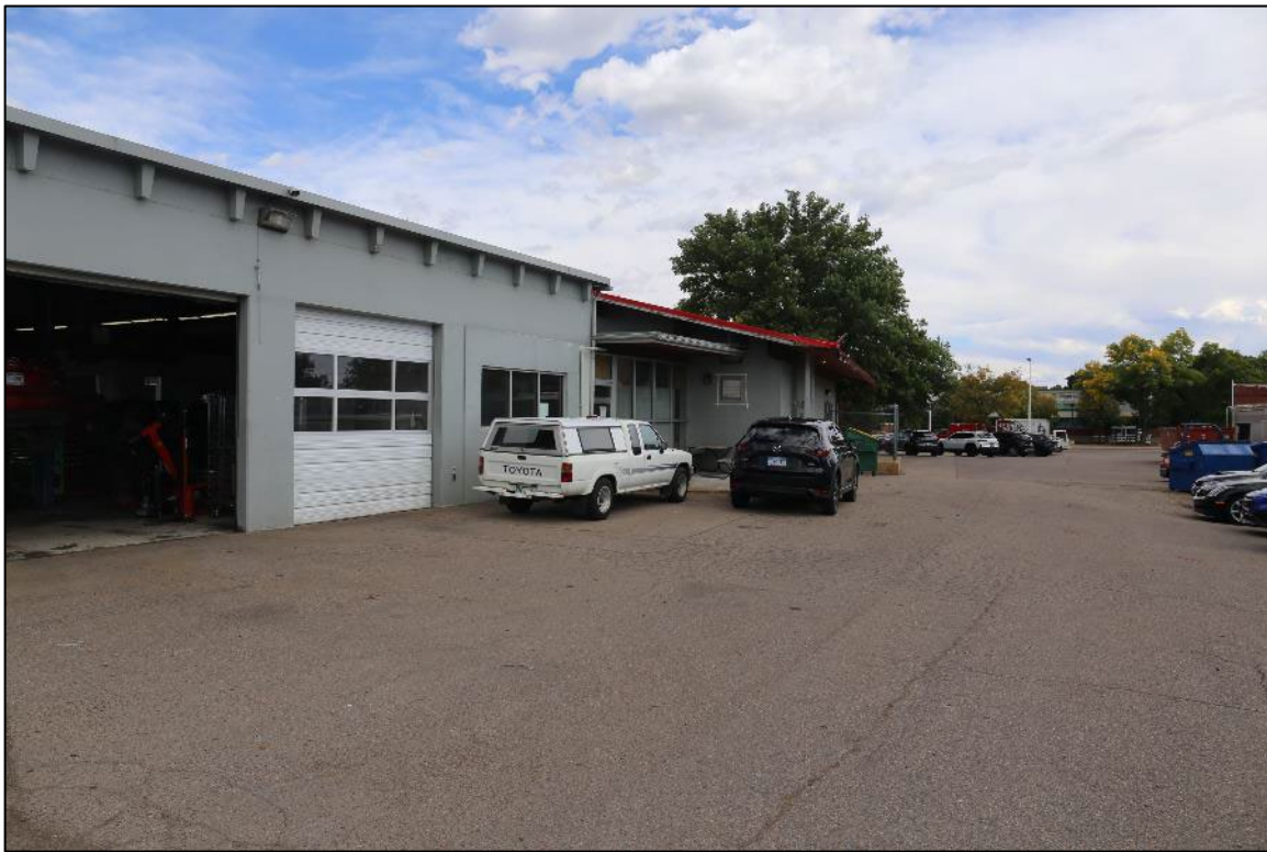
Figure 17: Feature 1, east end of south elevation. Note glass enclosed foyer between west and east portions of the building. (Image #7251, R. Shields, 10/3/2023).
