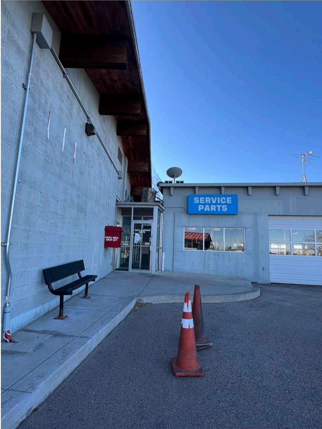
14. North Elevation - airlock entry of the service center, the customer service office, and the first of the bay doors. Image courtesy of BEE. 2024.
