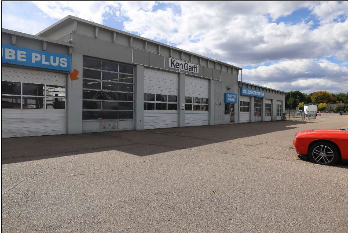
Figure 12: Feature 1, west half of north elevation, view southwest (Image #7224, R. Schields, 10/3/2023).
