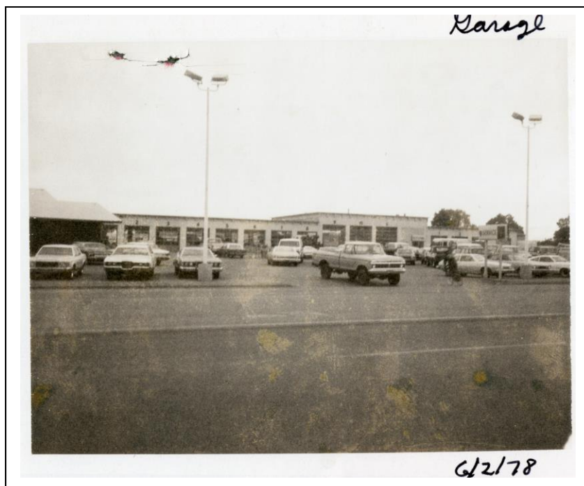
Ghents Motors (6/2/1978) Northern elevation of Service Bay Section. Photograph located Fort Collins Museum of Discovery. 2601SCol78_03.
