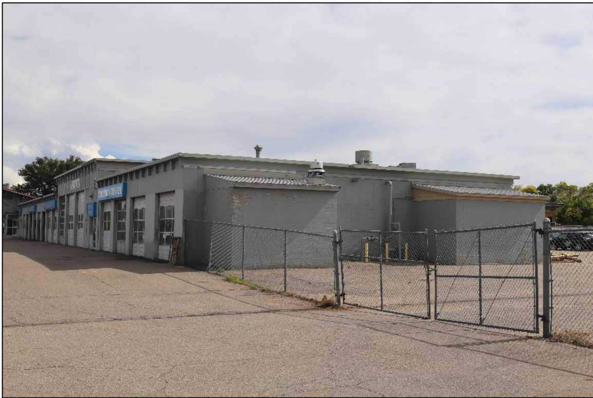
Figure 13: Feature 1, north and west elevations, view southeast (Image #7231, R. Schields, 10/3/2023).
