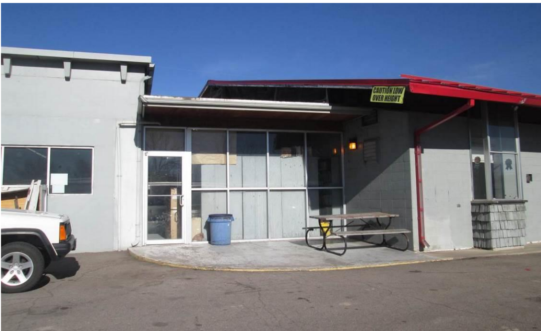
5LR.14283 – Spradley-Barr Foyer between Parts and Service Section and the Service Bay Section (Bldg. A) Southern elevation. Looking northwest. December 2017. Image 5LR.14283d.
