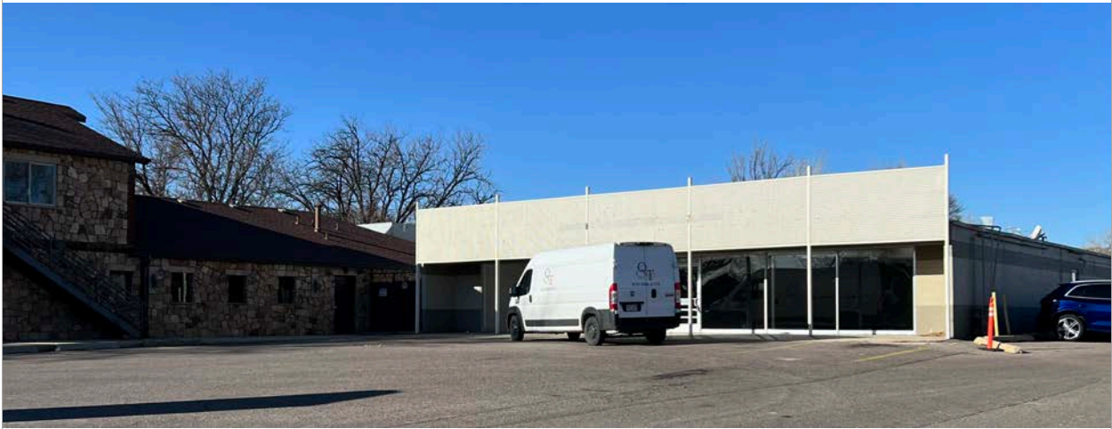
65. 2627 South College Ave. Property to the south of Car Dealership. Built in 1964, not eligible for landmarking per the City of Fort Collins Historic Resources Planning Map. Image courtesy of BEE. 2024.
