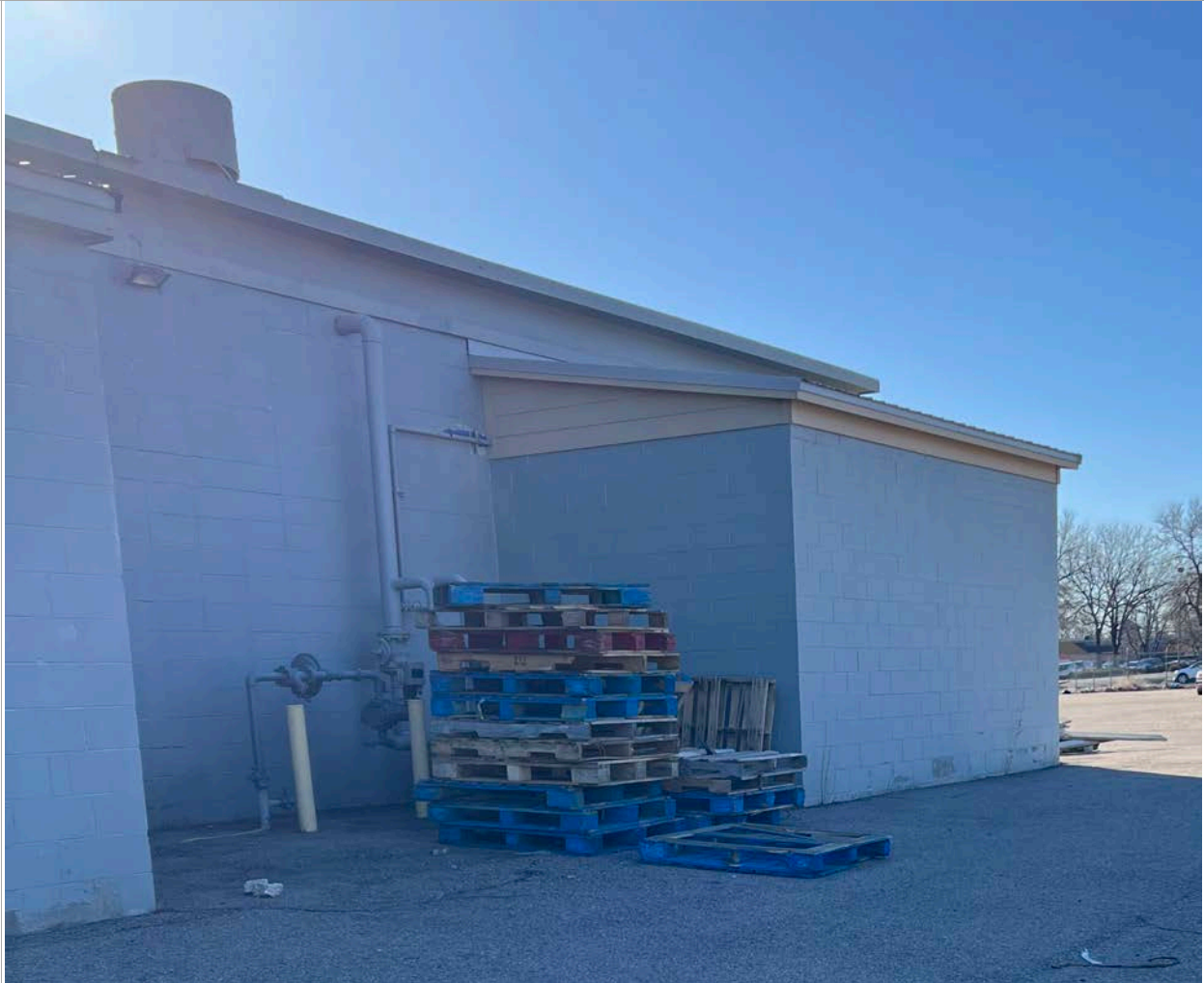
29. West Elevation - Detail at west, between storage sheds with gas meter. Image courtesy of BEE. 2024.
