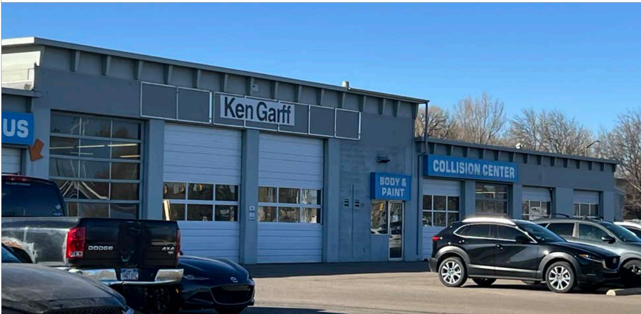
18. North Elevation - Service center, bays 9-11. Note the garage doors on bays 9 and 13 are original, all others have been replaced. Image courtesy of BEE. 2024.
