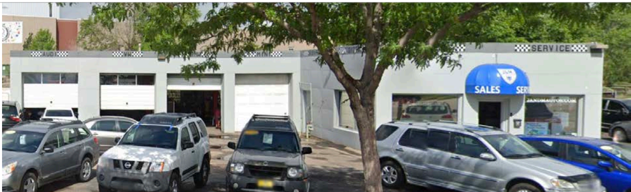
69. Saab Dealership, 425 North College Ave, date of construction unknown. Eligibility unknown. Image courtesy of Google Earth. 2024.
