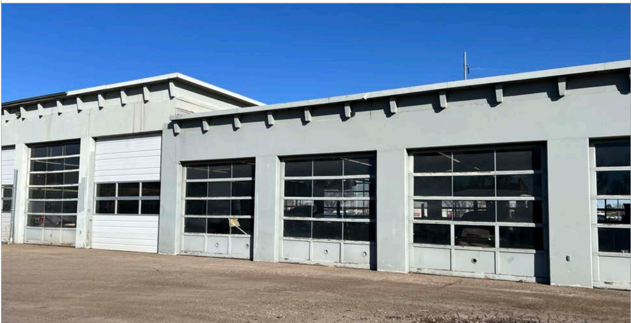
33. South Elevation - Service center, bays 5-11. Note more of the original garage doors on this elevation. Image courtesy of BEE. 2024.
