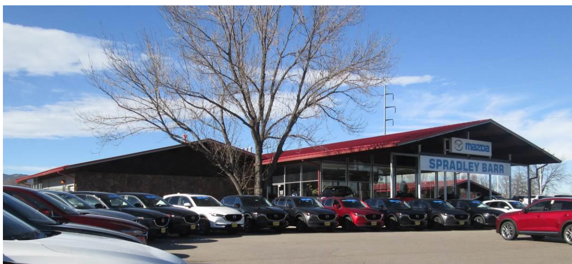
5LR.14283 – Spradley-Barr Showroom (Bldg. A) Eastern and southern elevations. Looking northwest. December 2017. Image 5LR.14283b.
