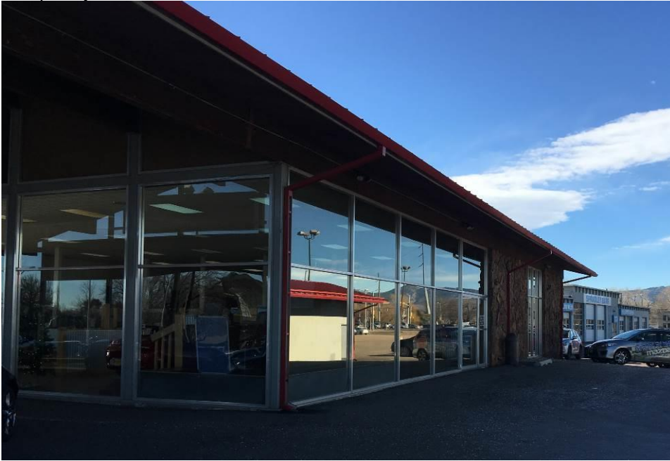
5LR.14283 – Spradley-Barr - Showroom (Bldg. A). Northern and eastern elevations. Looking southwest. December 2017. Image 5LR.14283h.
