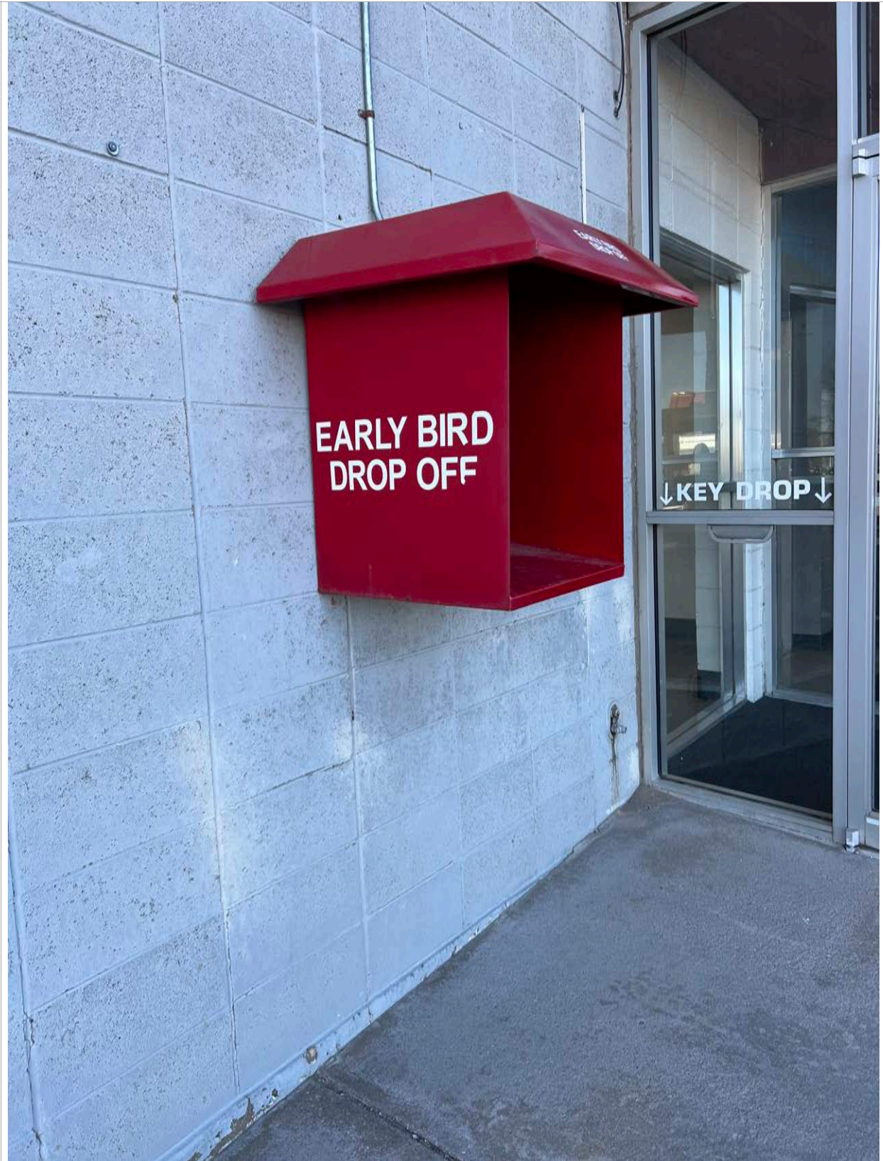
31. West elevation - Detail of key drop. Image courtesy of BEE. 2024.
