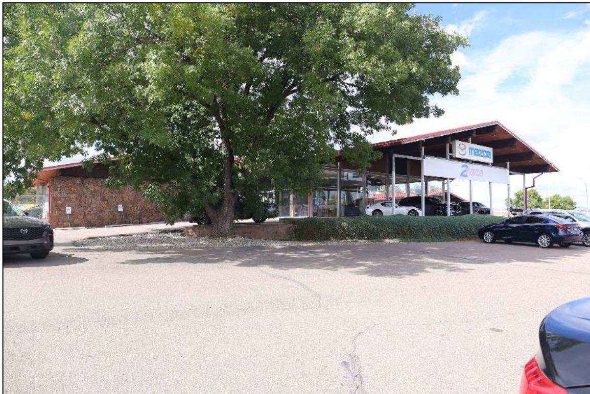
Figure 4: Feature 1, east-northeast elevation, view northwest (Image #7200, R. Schields, 10/3/2023).
