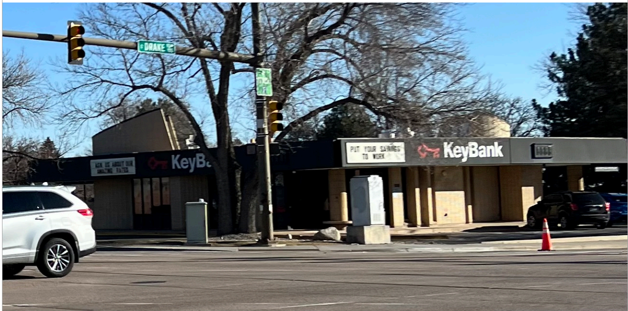
59. NE corner of Drake Rd. and S. College Ave. With an unknown construction date, the bank is deemed eligible for landmarking. Image courtesy of BEE. 2024.
