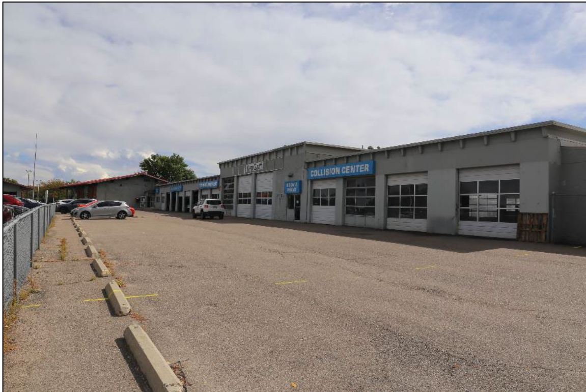
Figure 9: Feature 1, north elevation, view southeast (Image #7229, R. Shields, 10/3/2023).
