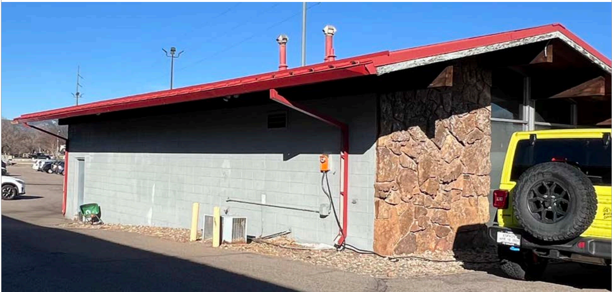
47. South Elevation - Small door at the service area. Image courtesy of BEE. 2024.
