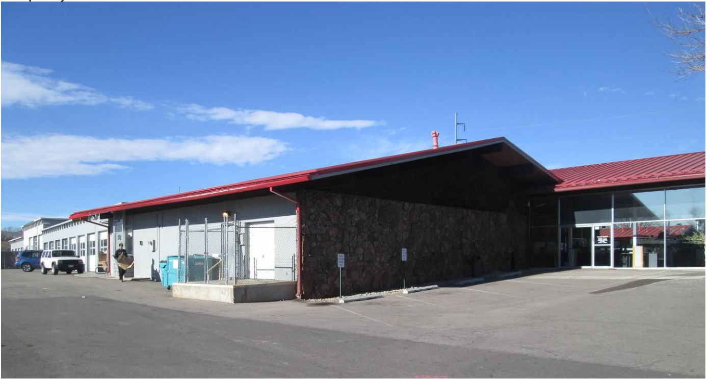
5LR.14283 – Spradley-Barr Showroom and Service Bay Section (Bldg. A) Eastern and southern elevations. Looking northwest. December 2017. Image 5LR.14283c.
