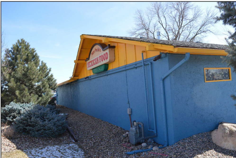
Photograph 12. The north wall from the west end. View southeast.
