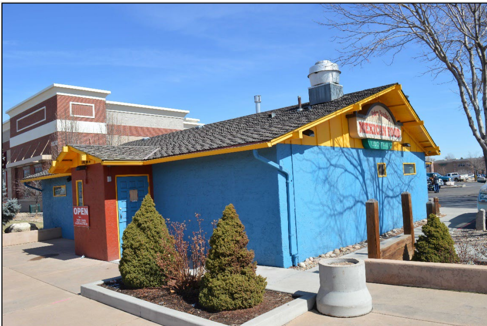
Photograph 4. Front and south wall. View northeast.
