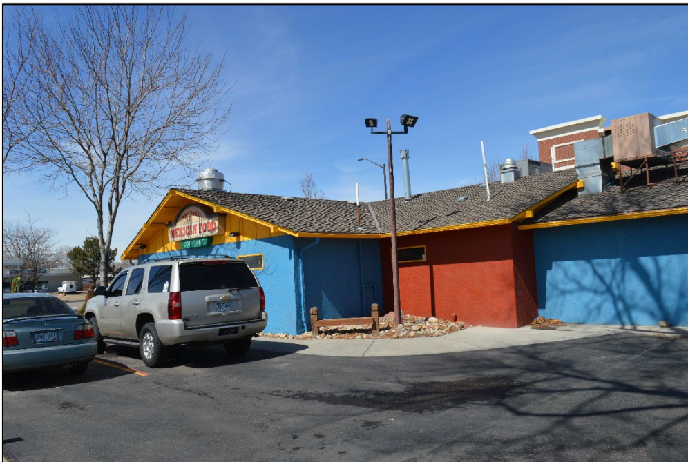
Photograph 8. The west part of the south wall. View northwest.
