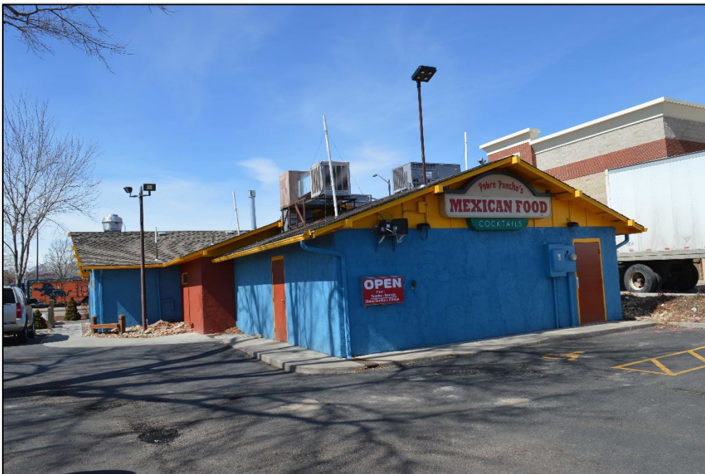
Photograph 10. The south and east (rear) walls. View northwest.
