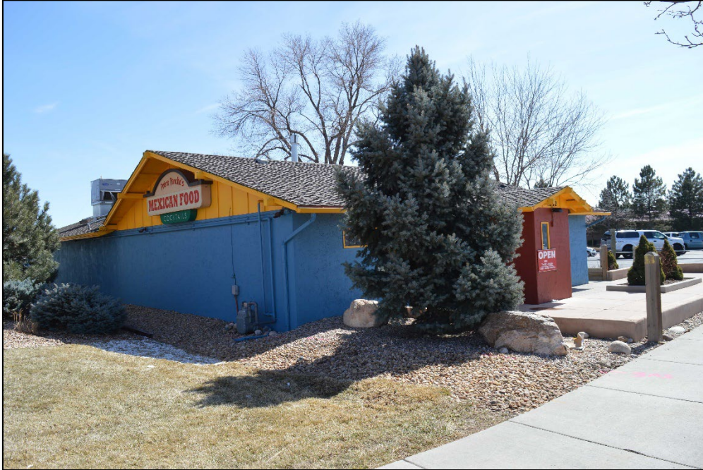
Photograph 13. North wall and. Front (west) wall. View southeast.
