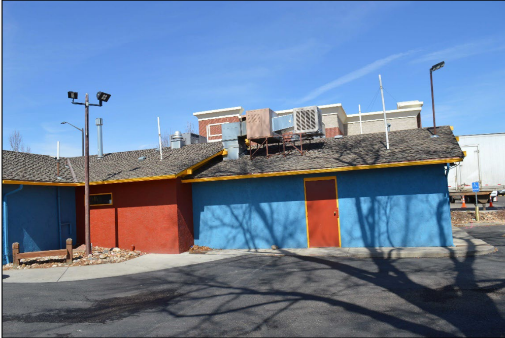
Photograph 9. The east part of the south wall. View north-northwest.
