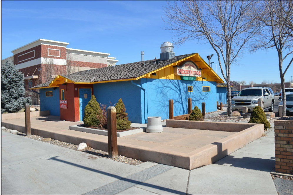
Photograph 3. The front (west) and south walls of the building and the patio area. View northeast.
