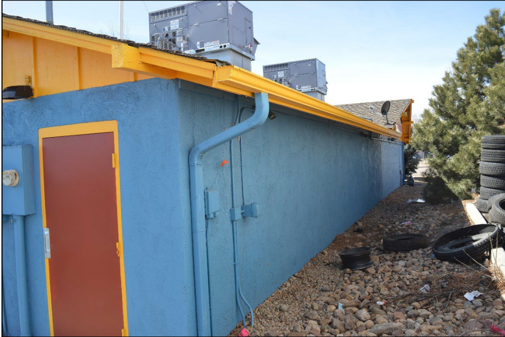
Photograph 11. The north wall from the east end. View west-southwest.
