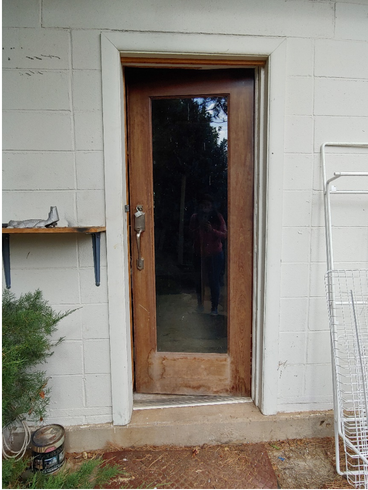
Photo 19 Garage southwest elevation - person door
