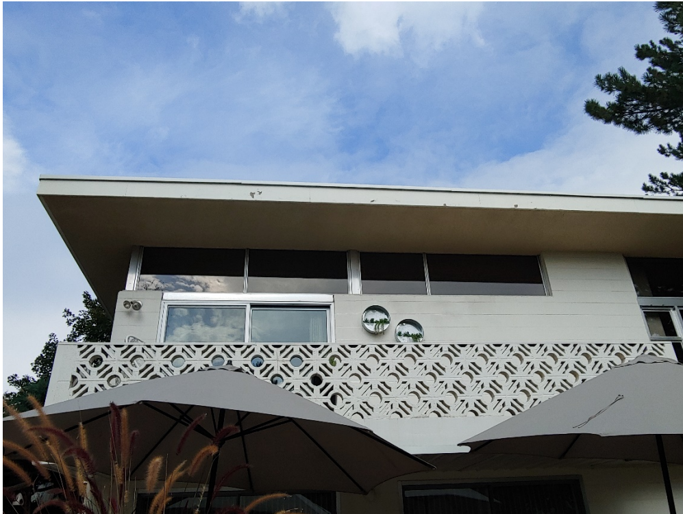
Photo 13 Southwest Elevation – Upper-level balcony, sliding glass door, and clerestory windows
