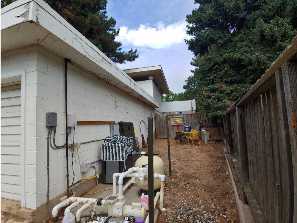
Photo 20 Southeast Elevation, wall, and fence
