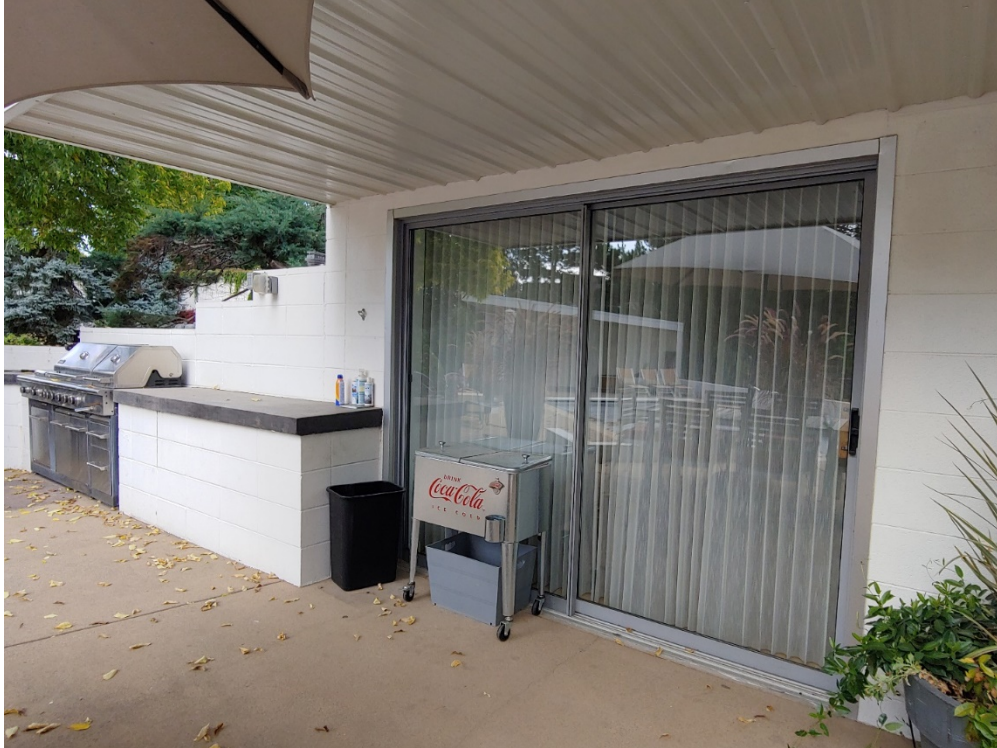
Photo 10 Southwest Elevation - Northmost sliding glass door and outdoor kitchen area
