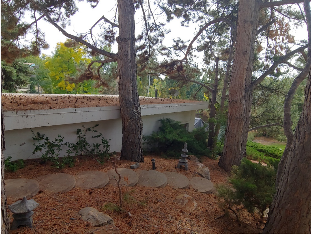
Photo 16 Garage northwest elevation
