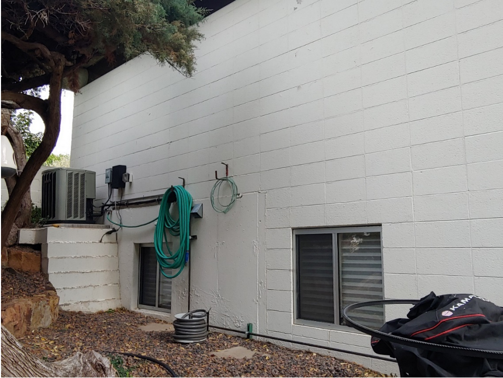
Photo 8 Northwest Elevation – Windows
