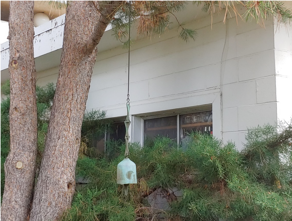
Photo 17 Garage northwest elevation windows
