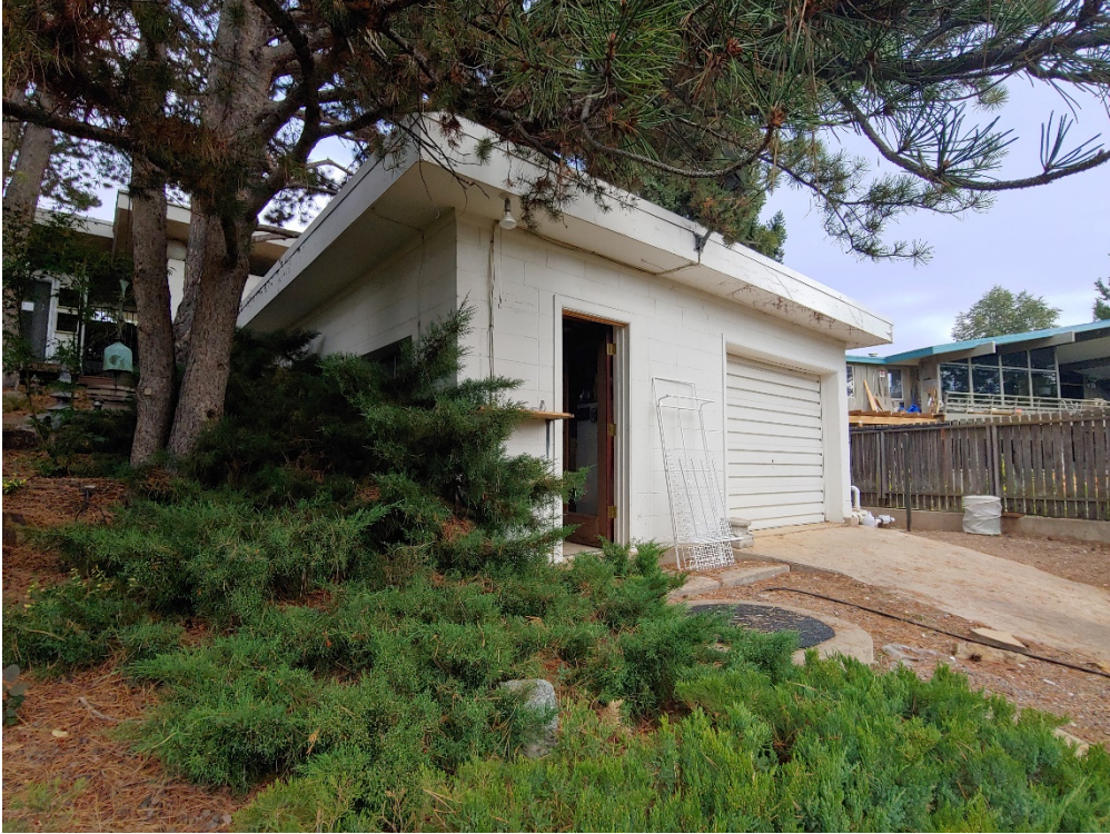
Photo 18 Garage southwest elevation
