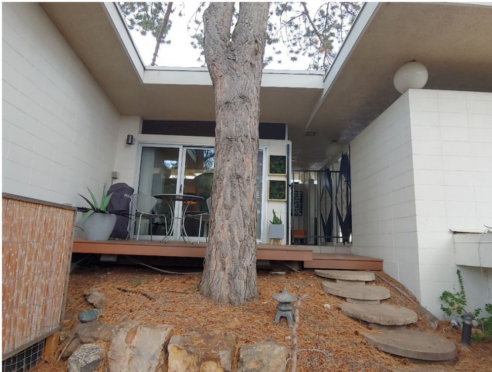
Photo 15 Southwest Elevation - Enclosed breezeway and gate to carport
