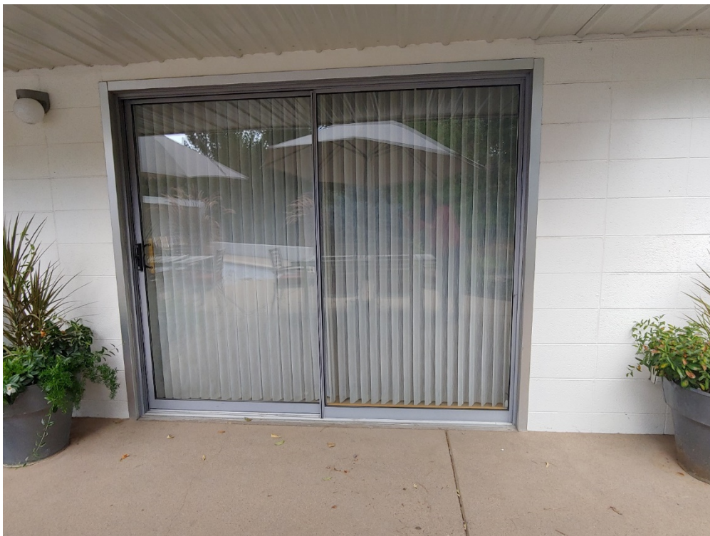
Photo 11 Southwest Elevation - Middle sliding glass door
