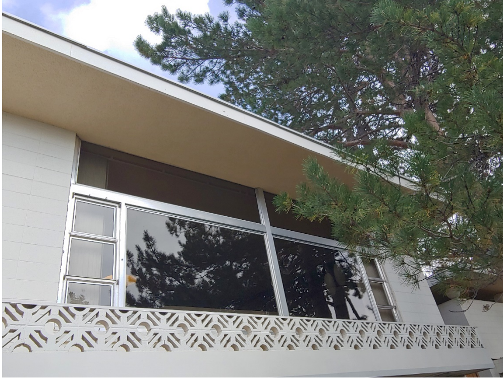
Photo 14 Southwest Elevation - Upper-level shorter balcony and windows
