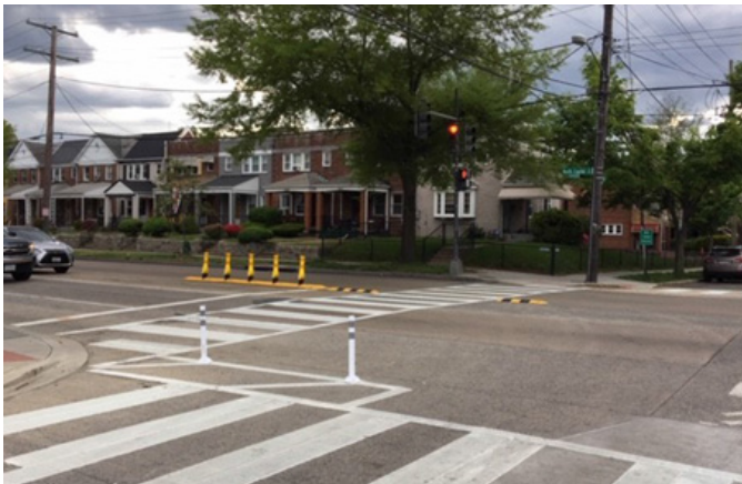
Figure 10: Flexible Delineators and Hardened Centerline to Control Turning Speed
