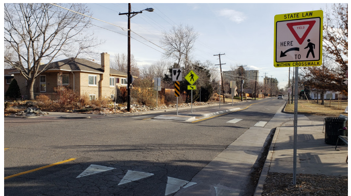
Advanced Yield Marking places in Advance of Crosswalk
