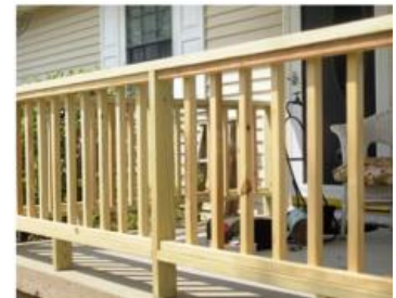
Front Porch & Handrail: Wood Pickets Color: Natural wood stain color
