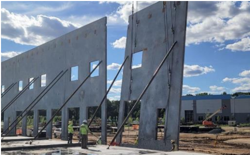
Exterior Siding: Tilt Up Concrete
