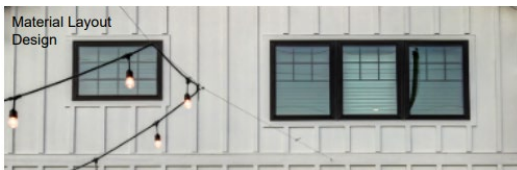
Exterior Siding: Board and Batten
