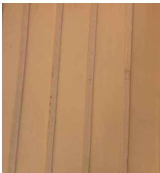
Exterior Siding: Board & Batton Siding
