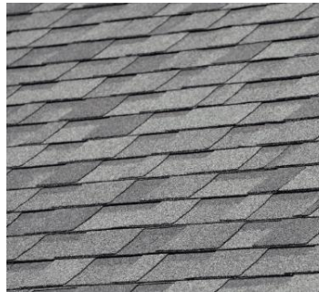
Roof: Fiberglass Shingles Roof
