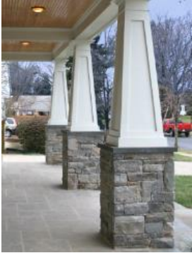
Columns: Stone Base Columns
