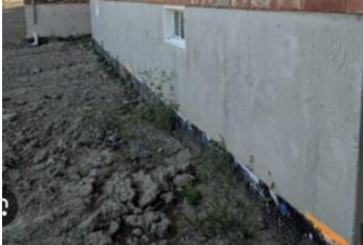
Foundation Wall: Exposed Concrete
