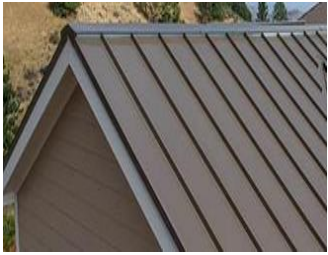
Roof: Standing Seam Metal Roof
