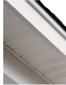
Soffit: Vinyl Soffit, Metal Wrap Fascia
