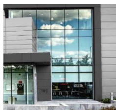
Windows: 1" Insulated Glazing (SolarCool SolarGray Reflective Surface on 1 st Surface, Clear on Inboard Surface)
