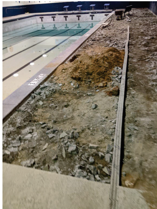
Photo 4 Review of slab removal
