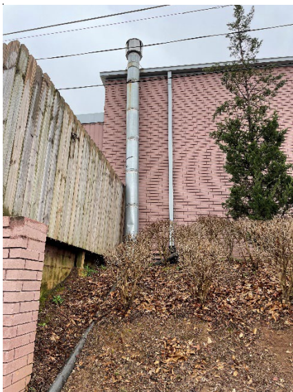
Photo 7: Exterior area E of equip room. View from E. 2/2023
