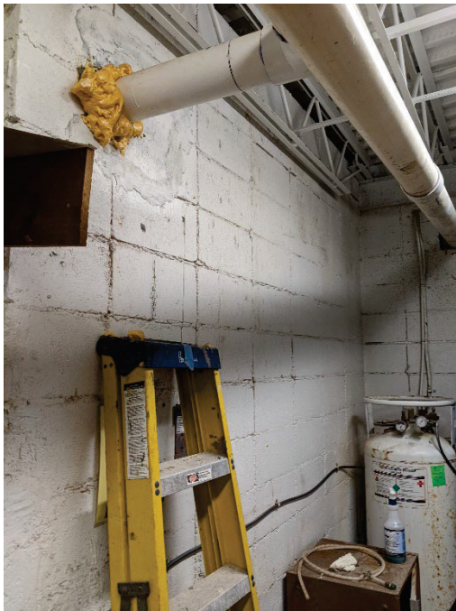
Photo 2 Southern Pool wall/Equipment Room Wall
