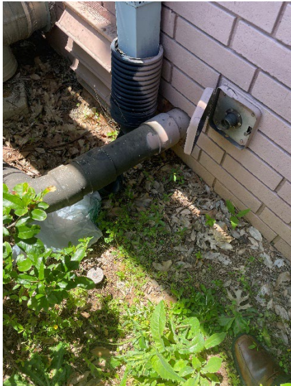
Photo 11: Area exterior to equip room. View from N. 5/2023
