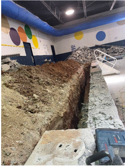
Photo 9: Excavated area N of pool. View from W. 5/2023
