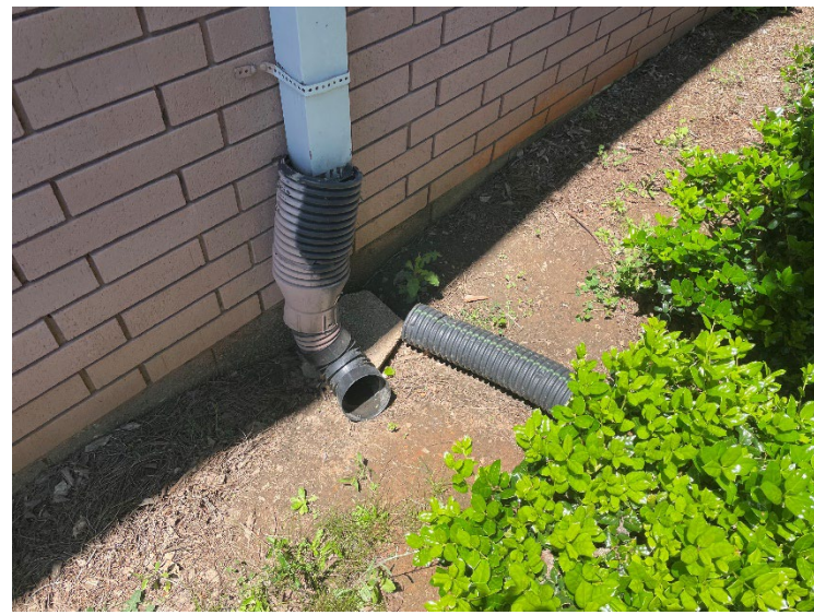
Photo 12: Down drain N of equip room. View from E. 5/2023
