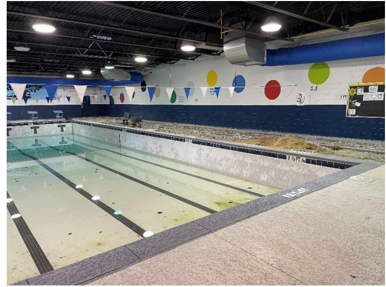
Photo 2: Demo area W of pool. View from NE. 2/2023
