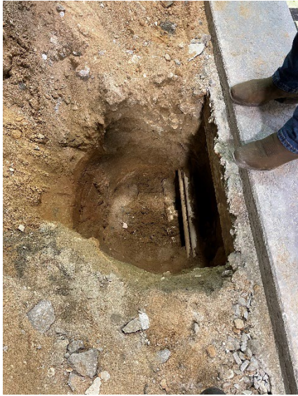
Photo 5: Excavation at inlet pipe leak. View from S. 2/2023
