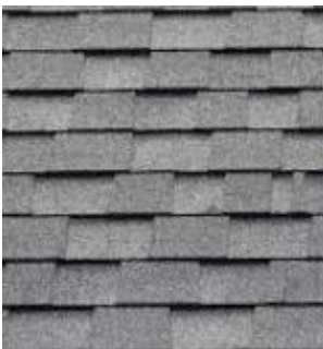
Roof: Architectural Shingles
