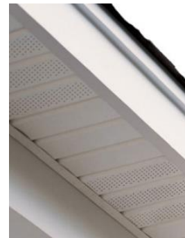
Soffit: Vinyl Soffit, Metal Wrap Fascia
