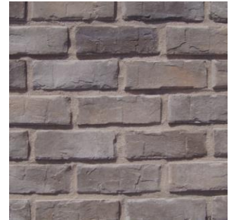
Exterior Siding: Brick Veneer Siding – Painted Brick Veneer
