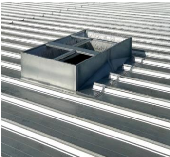
Roof: Mechanical Metal Roof.
