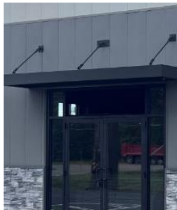
Canopy: Prefabricated Painted Metal: Color Black
