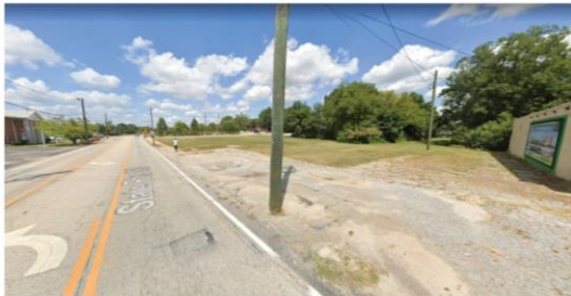
EXISTING MAIN STREET LOOKING WEST NEAR CARTERS CLEANERS & LAUNDRY
