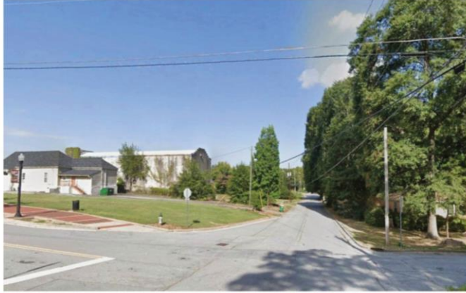
EXISTING HILL STREET LOOKING WEST AT THE INTERSECTION OF LAKE DRIVE
