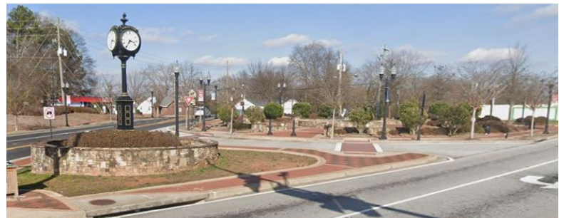
Roadway improvements along Main Street
