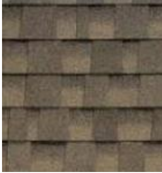
Roof Above Front Porch: Shaker Shingles
