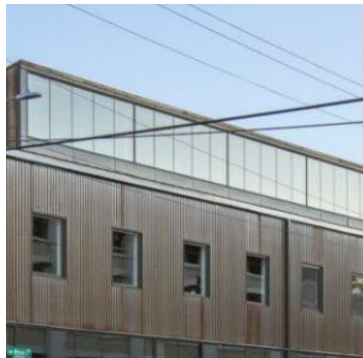
Windows: Clerestory Windows
