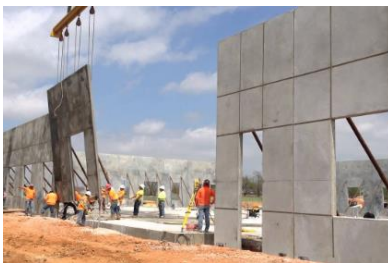
Exterior Siding: Concrete Tilt Panel
