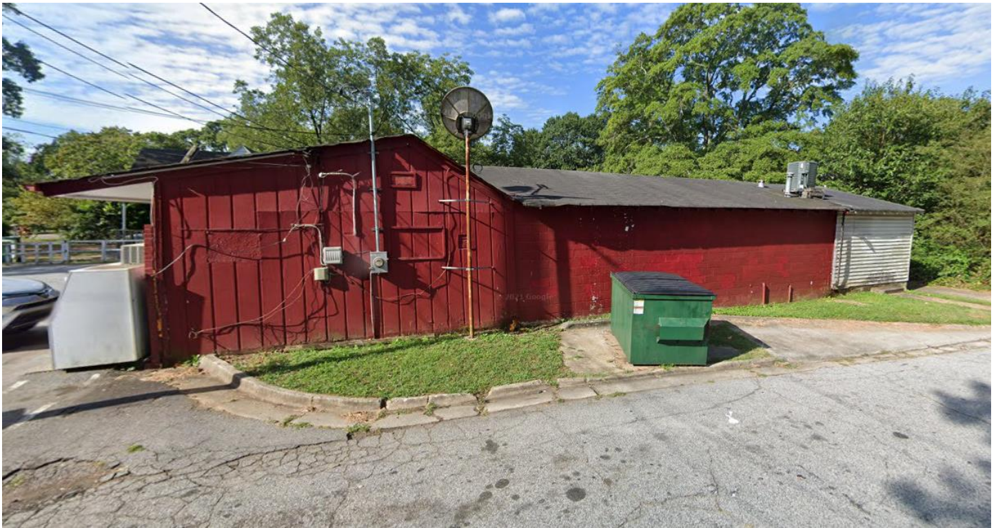
SIDE FAÇADE FACING BRIDGE AVE (MARCH 2022)
