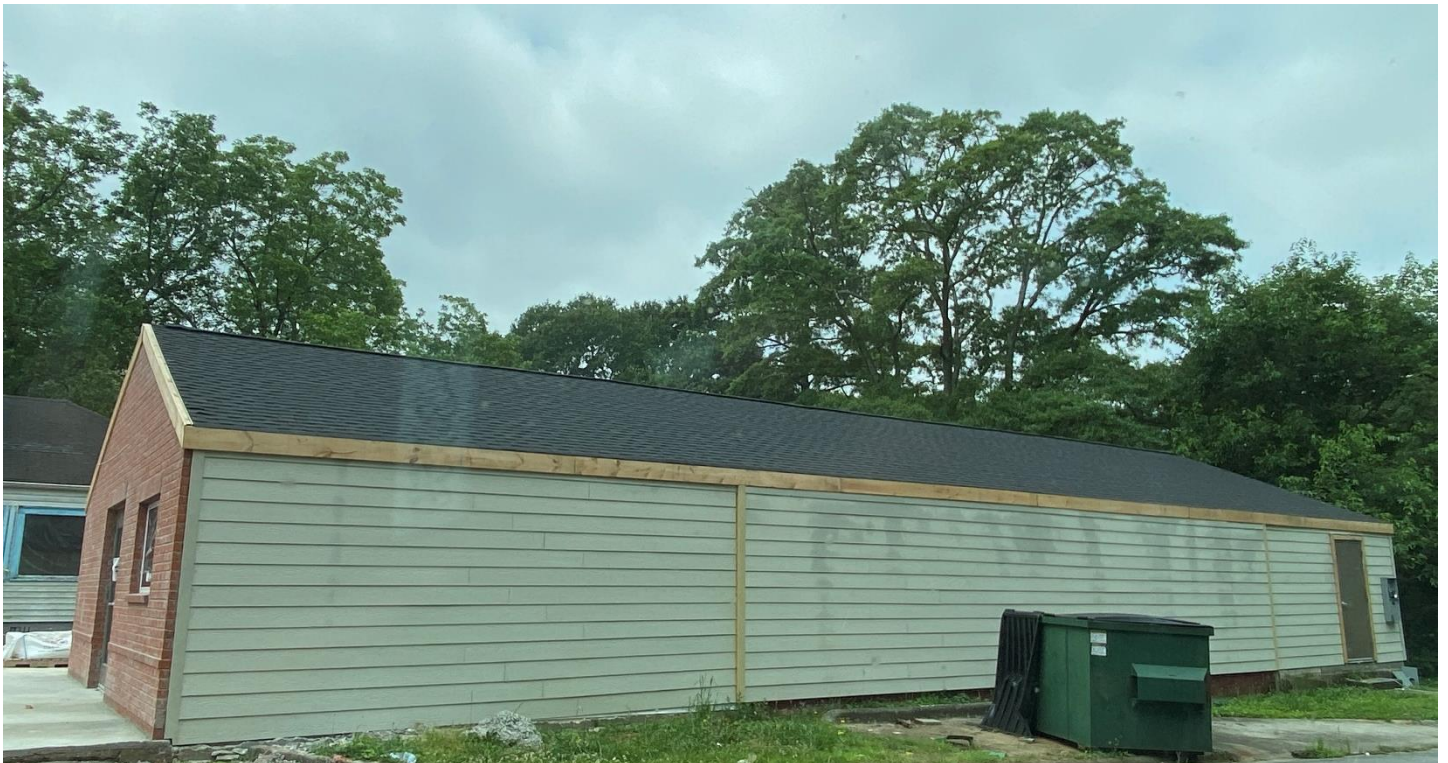
SIDE FAÇADE FACING BRIDGE AVE (JUNE 2023)
