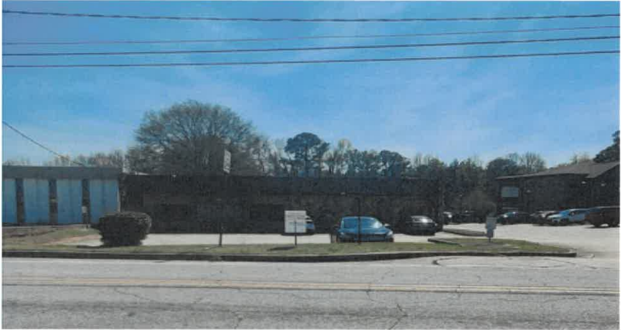
Vacant, Boarded Up Building
