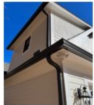
Rain Gutters & Downspouts: Five- Inch Aluminum
