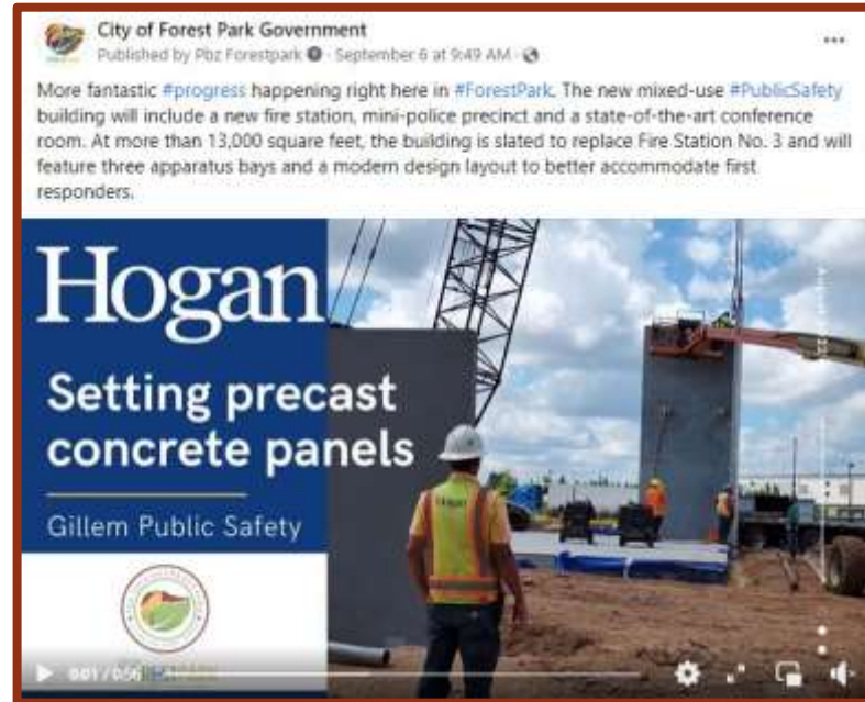
Construction on new Gillem Public Safety Building
