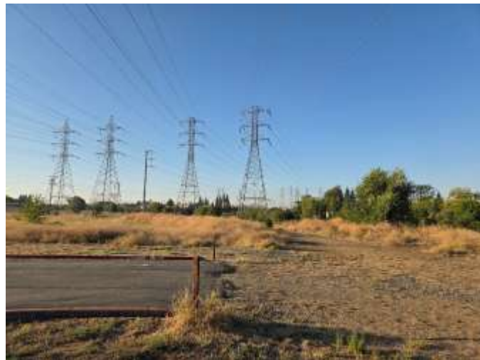
View of Subject Site
