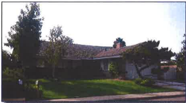
Example of California Ranch Architecture
