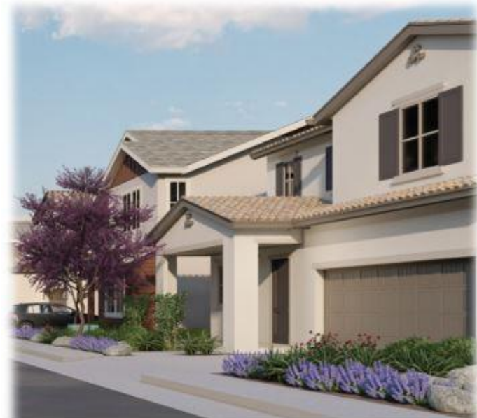
The large porch at Creekstone Plan 1 is a welcoming addition to the street scene.
