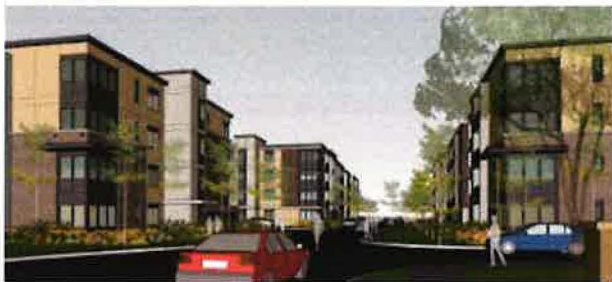
VIEW OF BUILDING 2, 3 & 4
