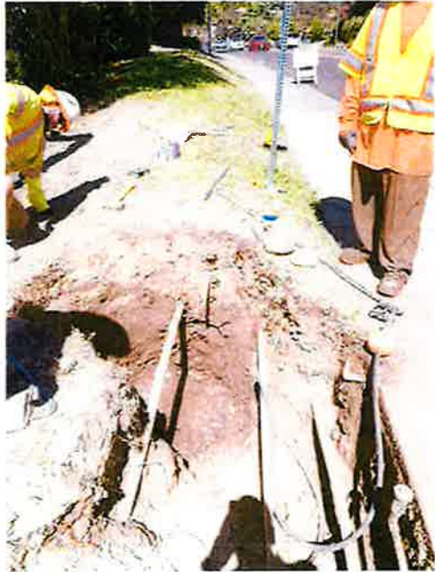
EXISTING BURIED MANHOLE PHOTO
