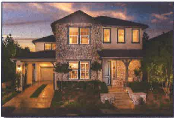
Porte Cochere with garage at rear of house
