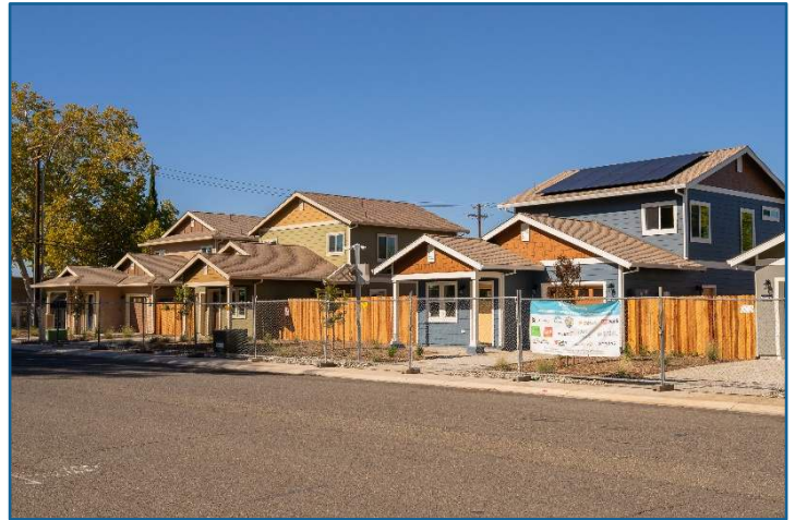
Newly Constructed Habitat for Humanity Homes
