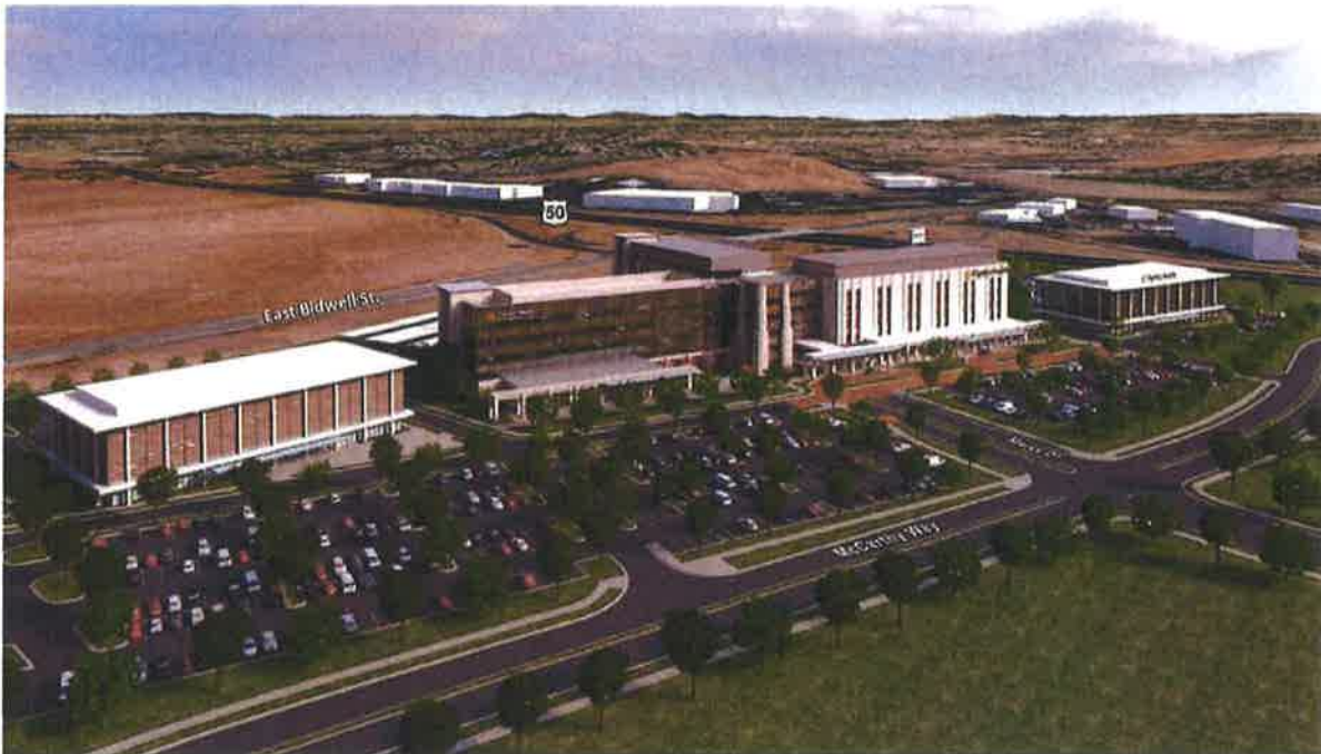
FIGURE 4: NORTHWESTERN VIEW OF ENTIRE MEDICAL CENTER
