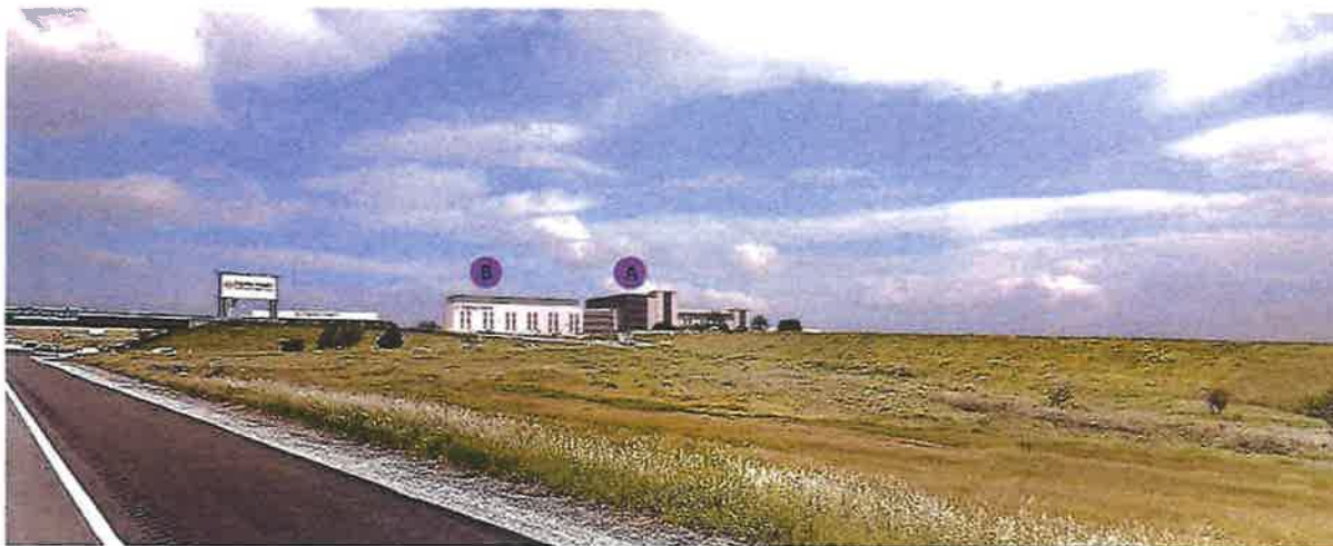
DISTANT READ PYLON/ FREESTANDING FREEWAY SIGN AND DISTANT READ BUILDING SIGNS VIEWED FROM EASTBOUND HIGHWAY 50
