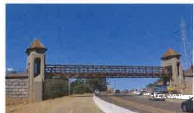
Some communities use arches or highly visible signage to signify a community gateway. The Johnny Cash Bridge serves as a gateway into Folsom.
