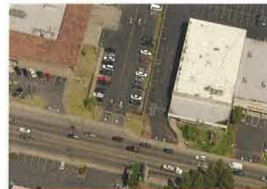
These two strip malls in another community have four driveways nearly adjacent to each other. This creates an unsafe and unpleasant environment for pedestrians and drivers.
