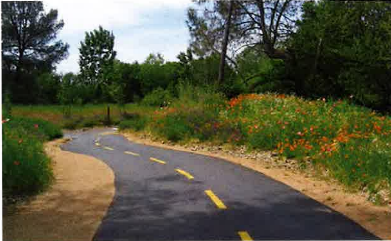
Centerline striping along a shared use path in Folsom helps to communicate that users should expect travel in both directions and encourages users to travel on the right and pass on the left.
