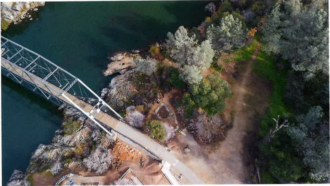
View of the Historic Truss Bridge and existing river overlook area from above
