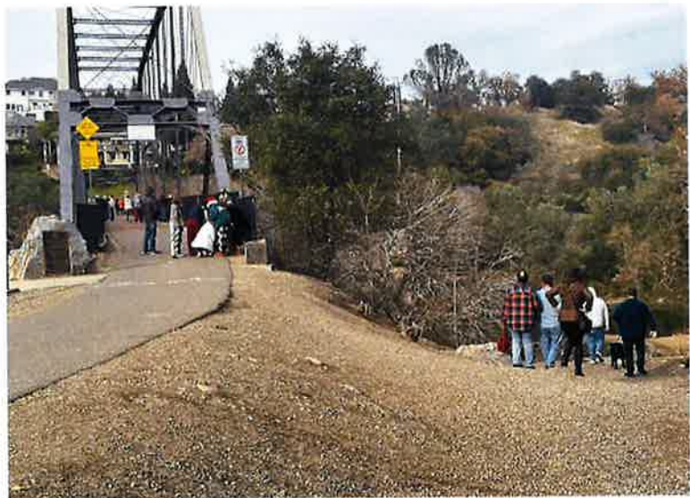
The area around the Truss Bridge is frequently congested with a multitude of trail users and people seeking access to the water
