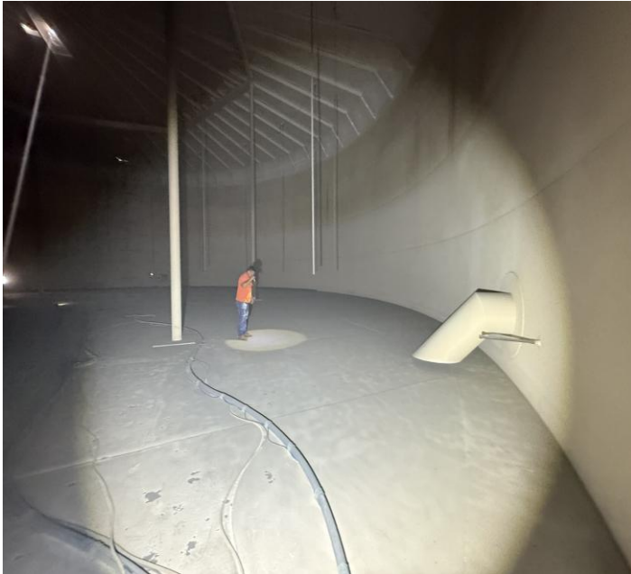
Interior floor of the Foothill Tank. Picture #3
