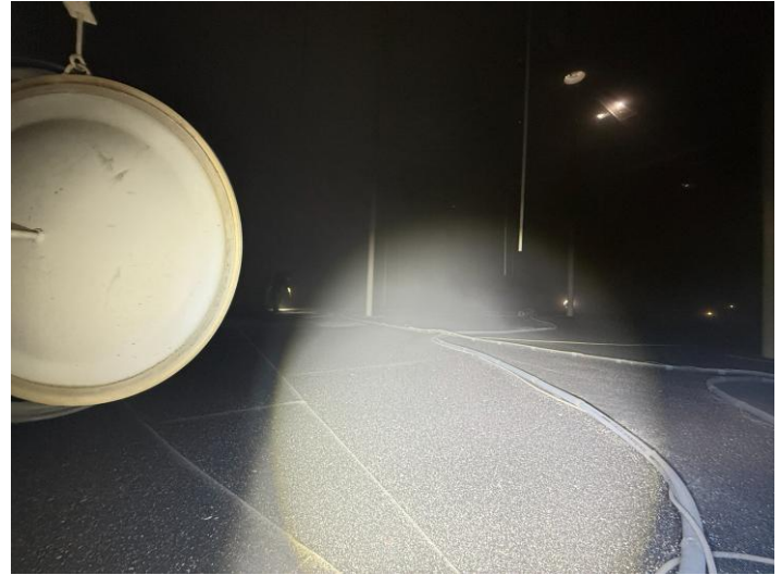
Sweep blasting operations being performed on the interior floor. Picture #2
