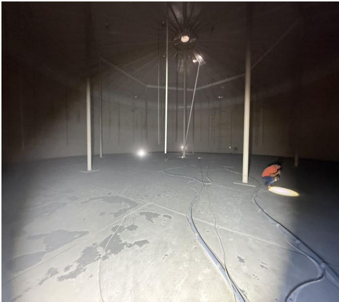
Interior floor of the Foothill Tank. Picture #1
