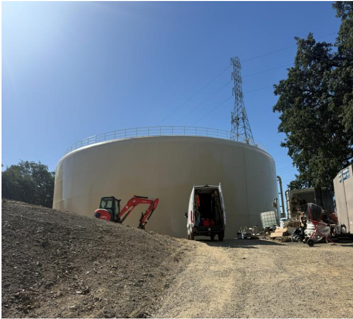
Tower Tank Project.
