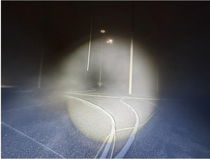
Sweep blasting operations being performed on the interior floor. Picture #1
