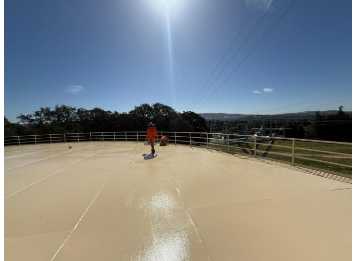
ESM crew members performing 2 nd finish coat application to exterior roofs handrails.
