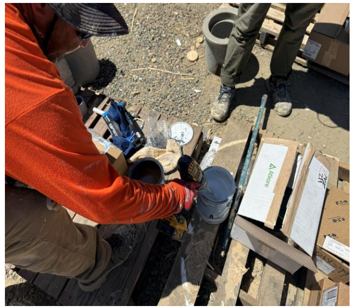
Part A & B of Macropoxy 646 being pre-mixed prior to beginning mixing operations.
