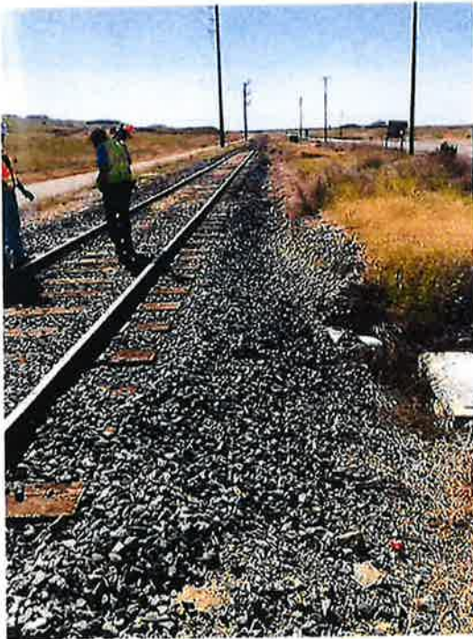
Shoulders cut off ties for drainage create a tripping hazard in the walkway.
