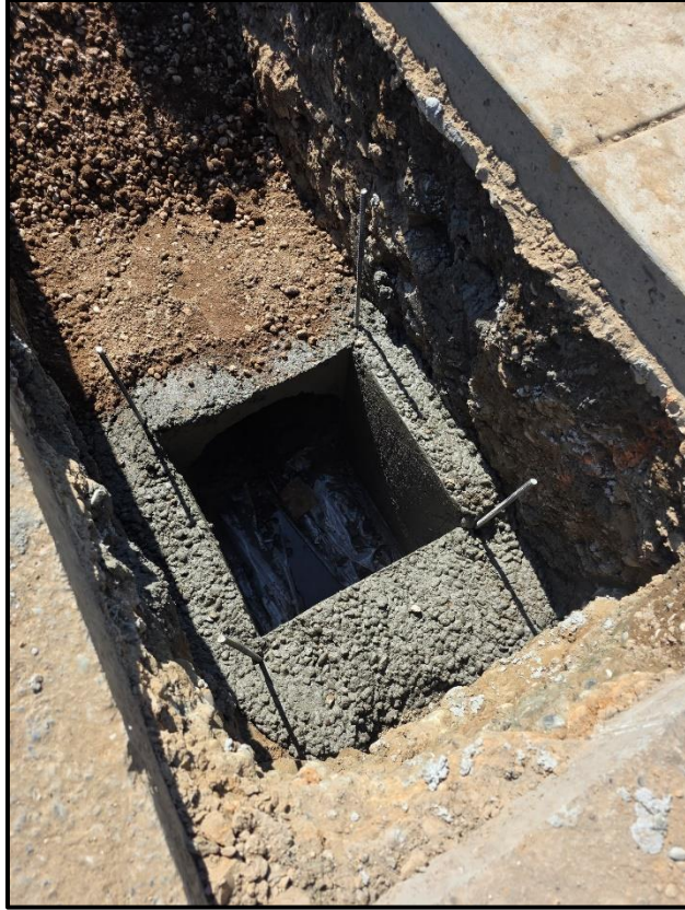
Cast-in-place junction structure connecting new 24-inch storm drain with existing
