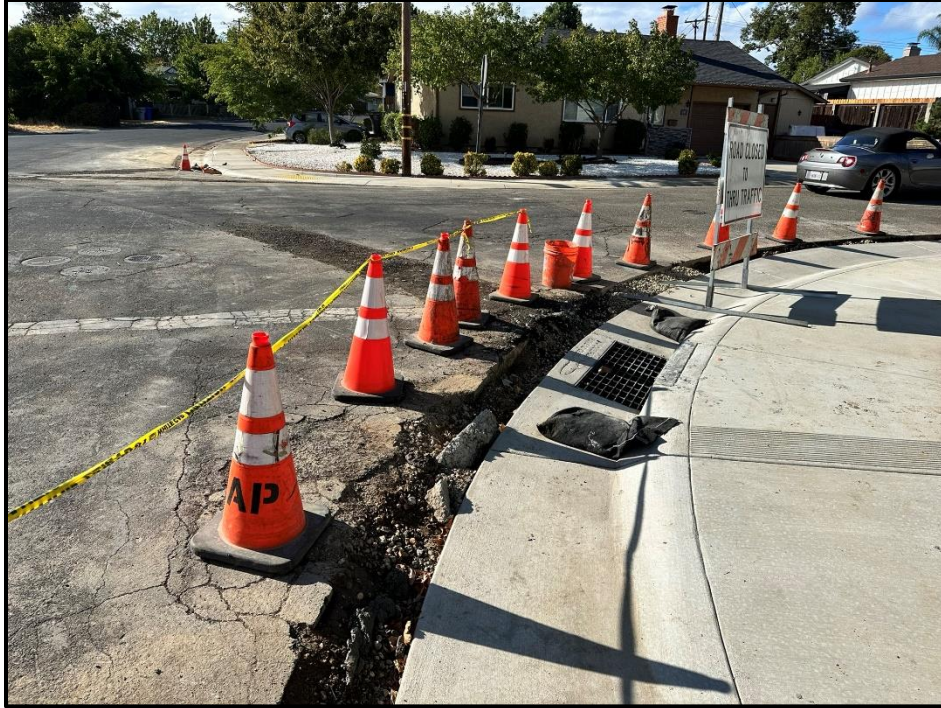
Area of additional asphalt work at northeast corner of intersection, looking west
