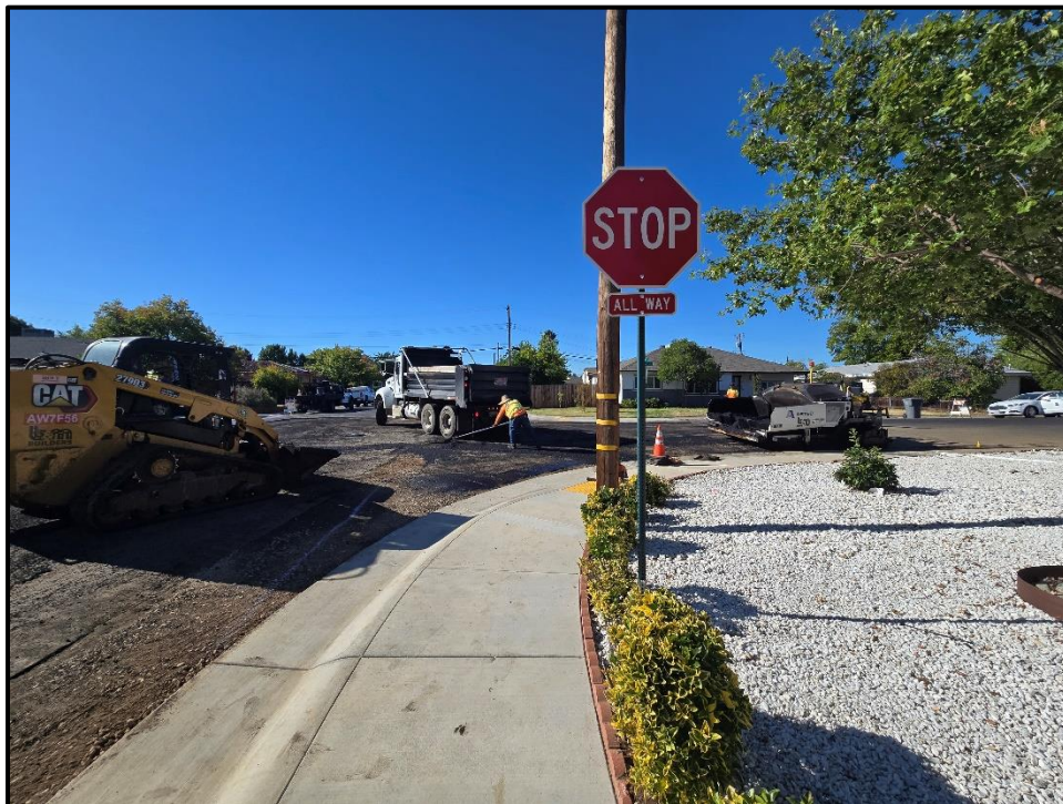
Area of additional asphalt work at northeast corner of intersection after grinding operations, looking west
