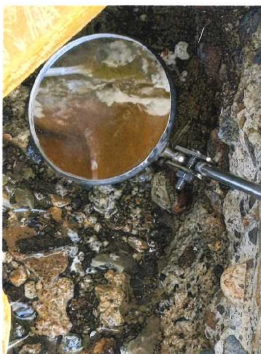
Discharge Rear Face Flange Leak (Feed Pumps)
