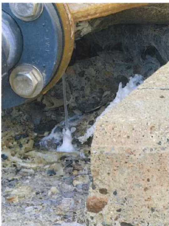
Discharge Rear Face Flange Leak (Feed Pumps)
