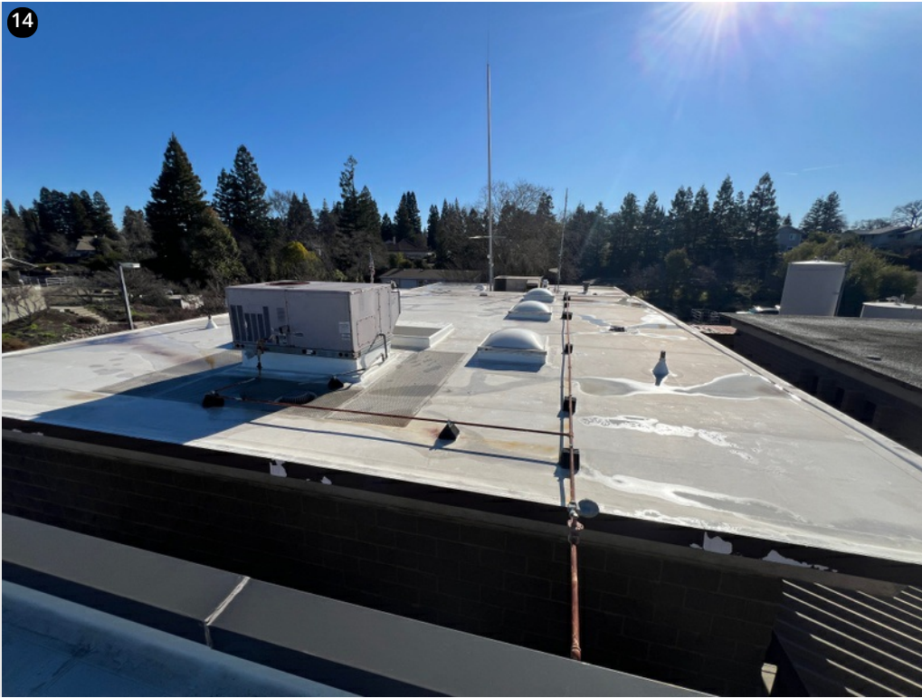
Upper main roof.
