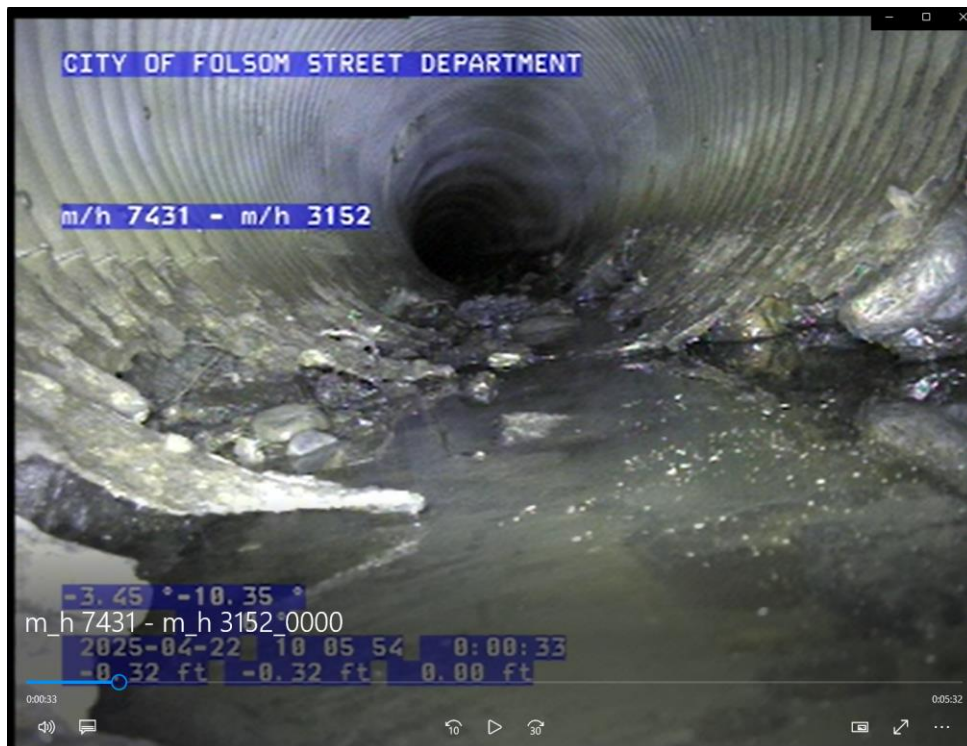
Glenn Drive storm drain - inspection showing failing storm drain
