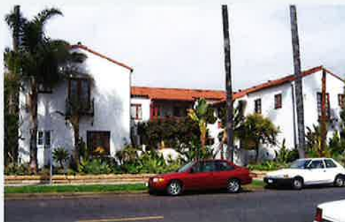
Above: House-scale courtyard building 8 units; 31.7 du/ac. Building back bar 84 x 32, wings coming to street 31 x 25, courtyard 30 x 36; 2 Stories
