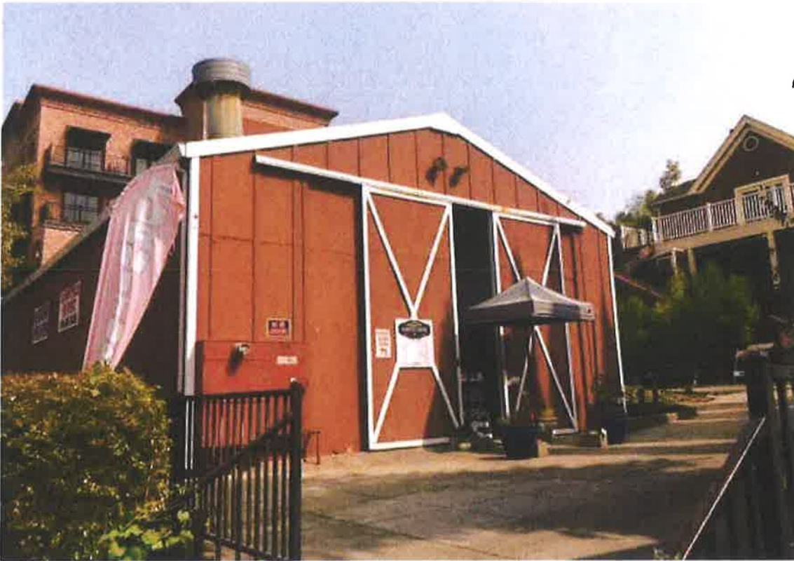
FIGURE 4: COMMERCIAL BUILDING AT 608 ½ SUTTER STREET
