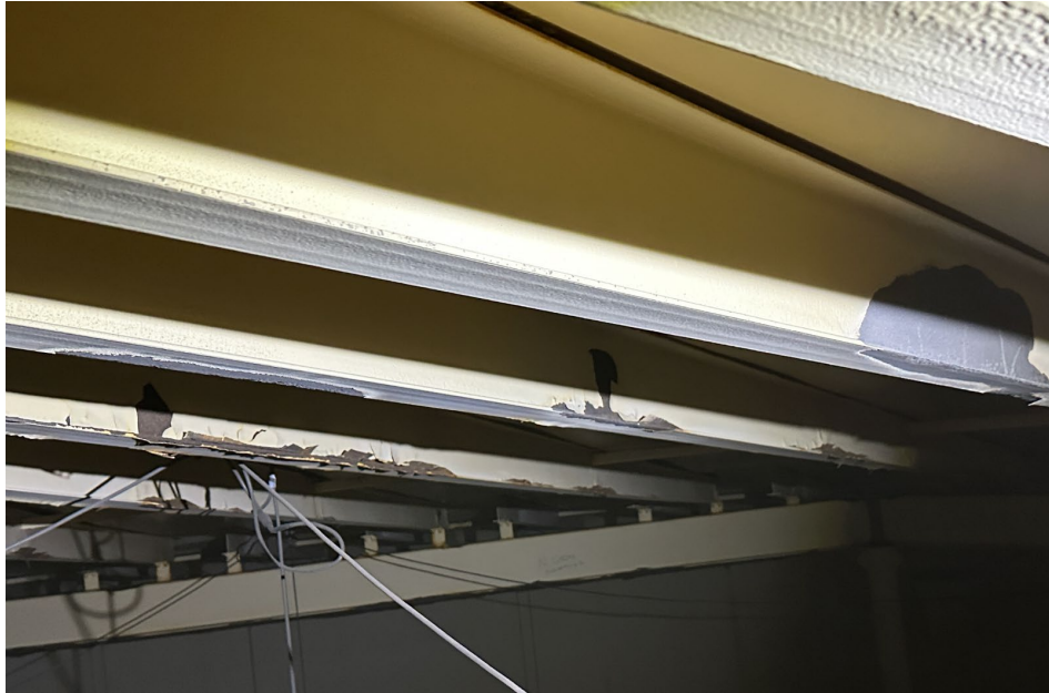
W8x10 Beam Deterioration
