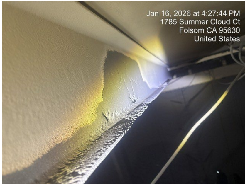
9. Photo No. 9 – Foothills Tank No. 1 rafter bottom flange corrosion
