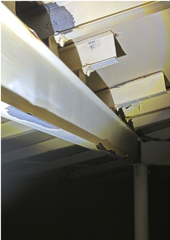
W16x26 Girder Flange Corrosion
