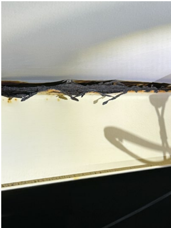
W8x10 Top Flange Corrosion Paint Showing Primer Debonded from Steel
