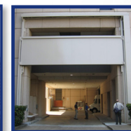
Vertical Lift Flood Barrier
